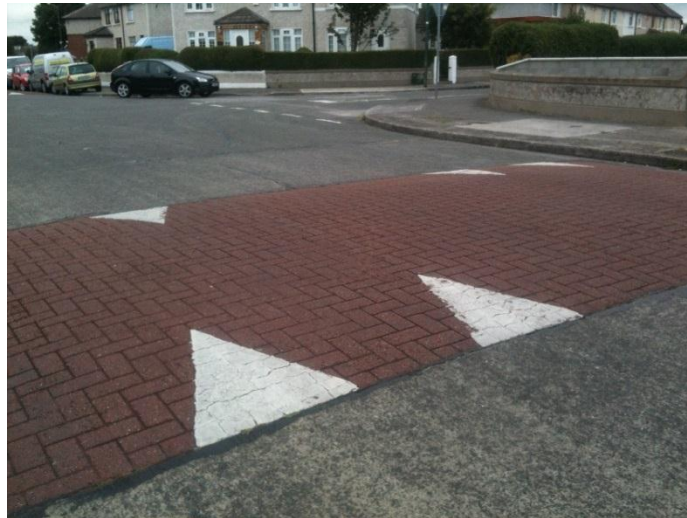
Figure 4.2 Example of a Road Hump in UK
