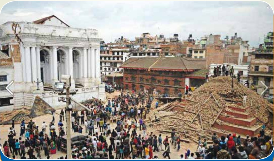
Photo: Kathmandu Durbar Square, a Cultural Heritage Damaged by Gorkha Earthquake
