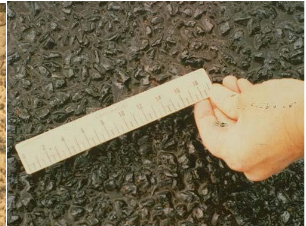
Figure 6: Chip Seal Before and After Fog Seal
