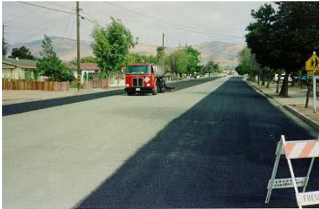
Figure 2: Fog Seal Application
