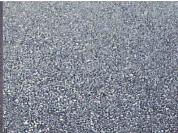
Figure 5: Suitable Surface, Open Graded HMA
