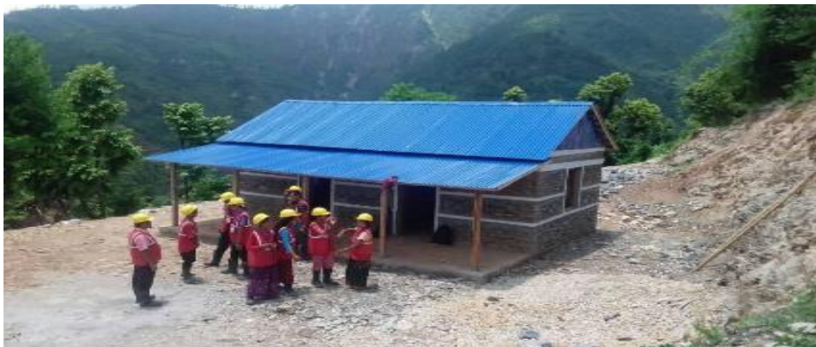
Fig.3: Demonstration House Construction; May 2018
