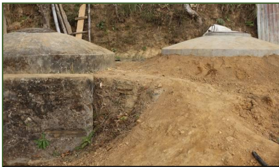
New water tank constructed under the GRR program
