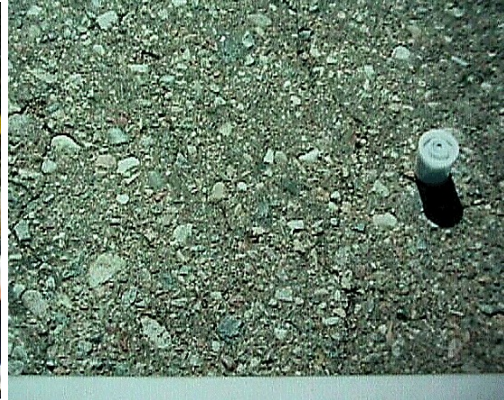
Figure 3: Suitable Surface, Heavily Aged Dense Graded HMA
