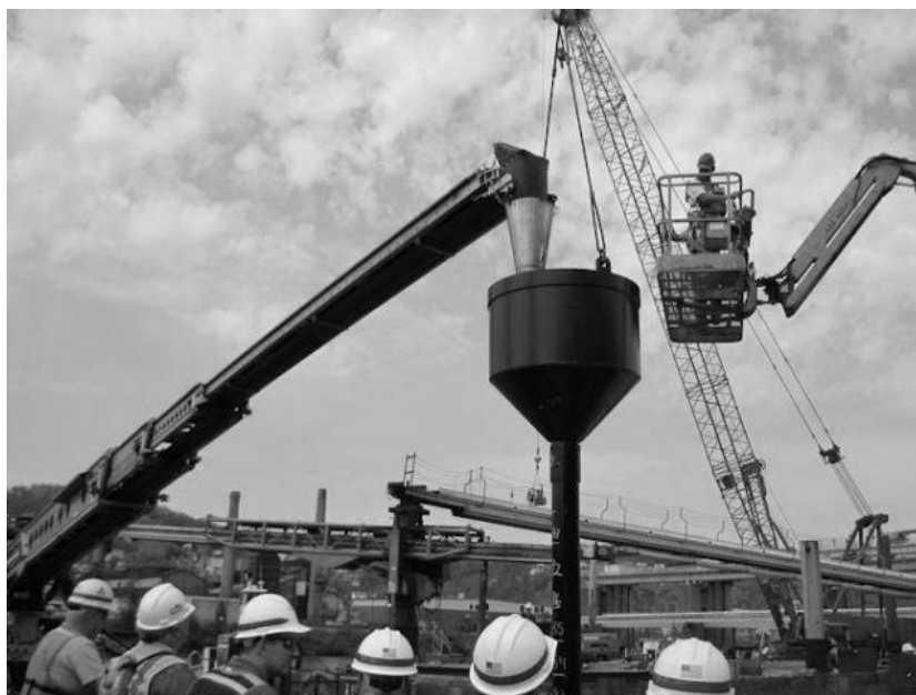
Figure 3.1 Tremie Concreting Method
