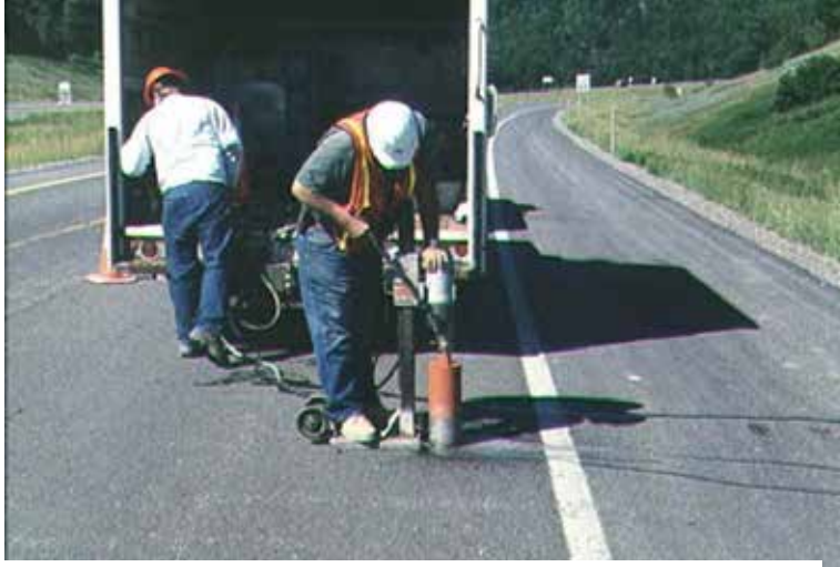
Figure 6.4 Coring hot mix asphalt
