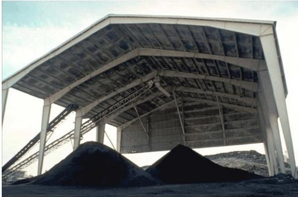
Figure 4.8 Covered aggregate stockpiles.
