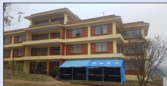
Quarantine center at Kharipati, Bhaktapur
