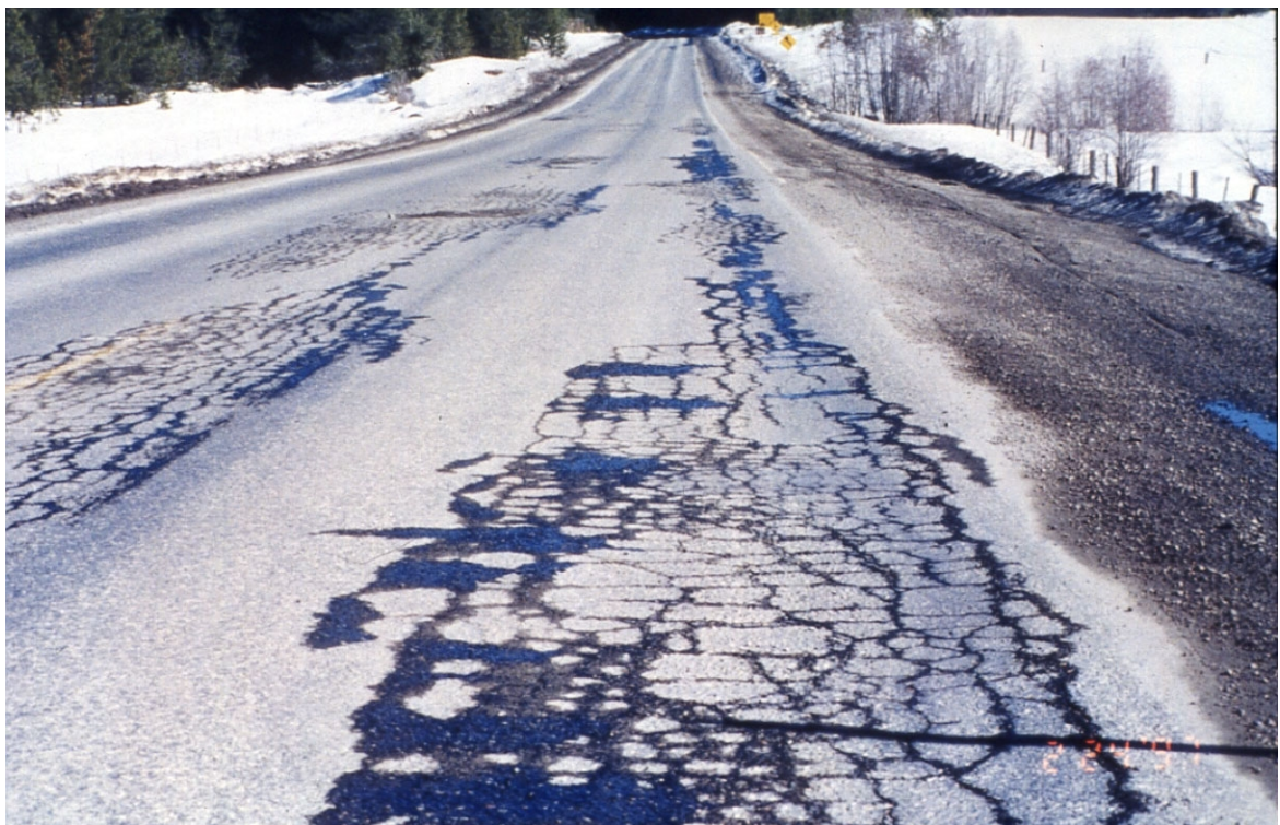
Figure 9.4. Freeze-thaw damage.
