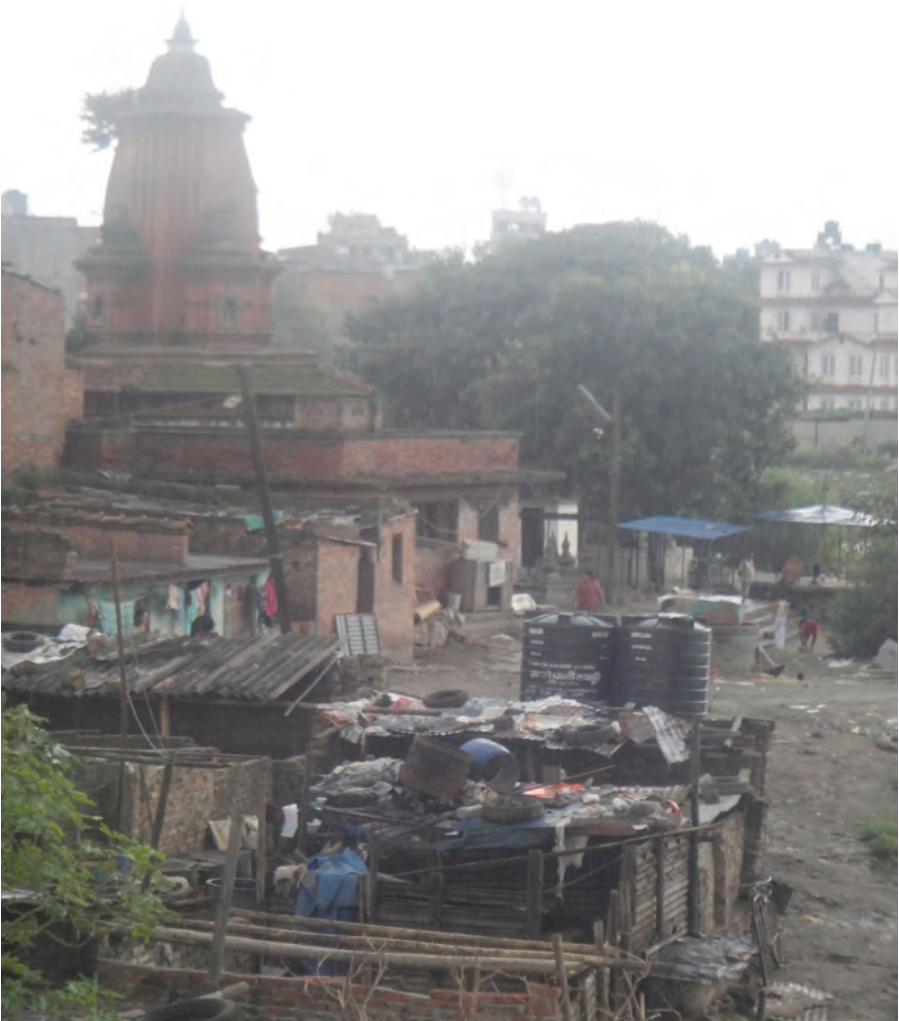
The condition of temples along the riverbanks in the Kathmandu Valley is deteriorating due to encroachment and inadequate solid waste management.
