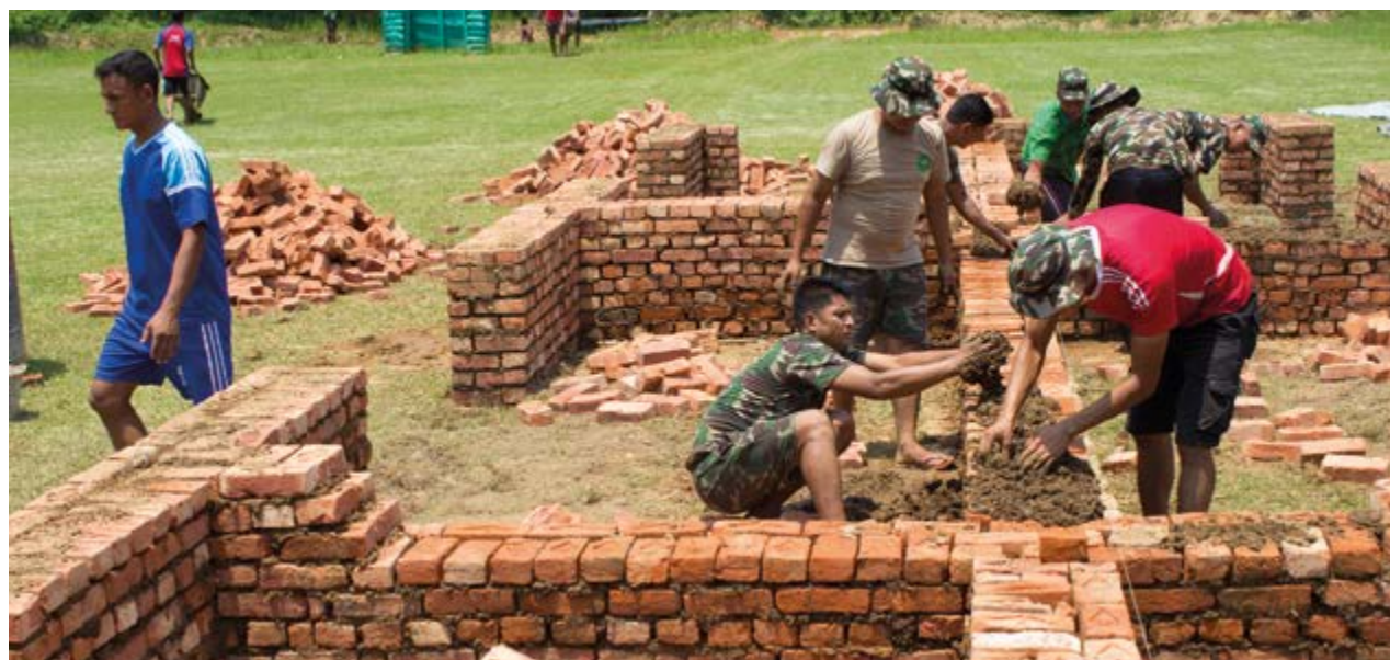
Construction of the furnace using brick and mud
