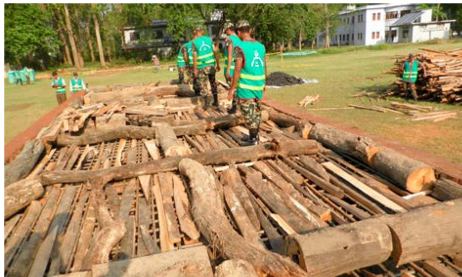
Laying wooden logs above MS bar
