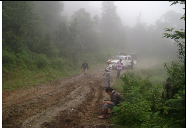
View of some existing roads
