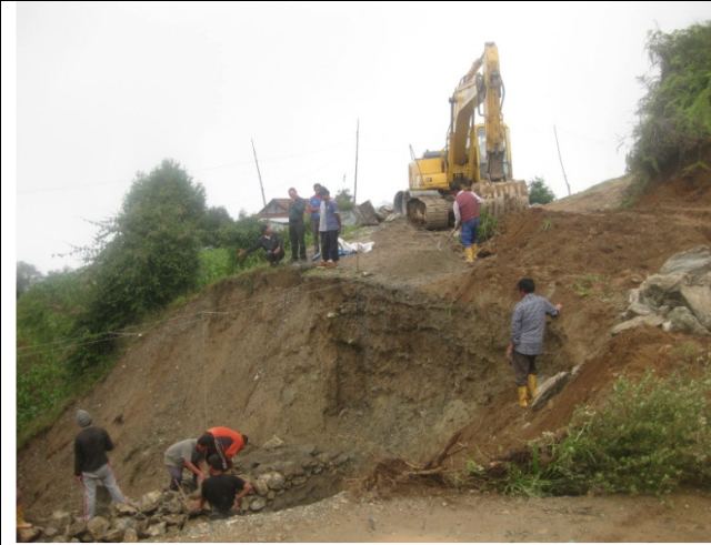
View of some existing roads
