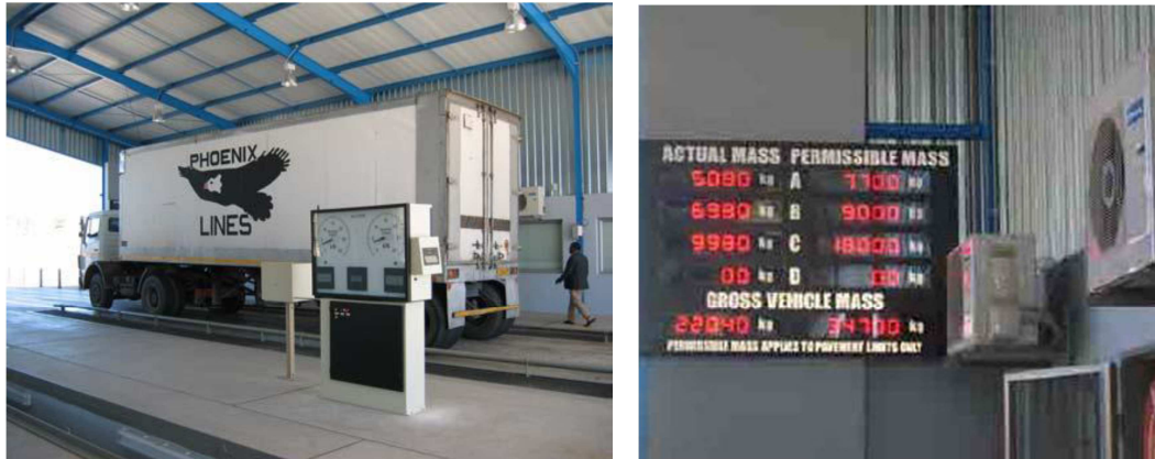
Figure 2.3 Multi-deck Weighbridge
