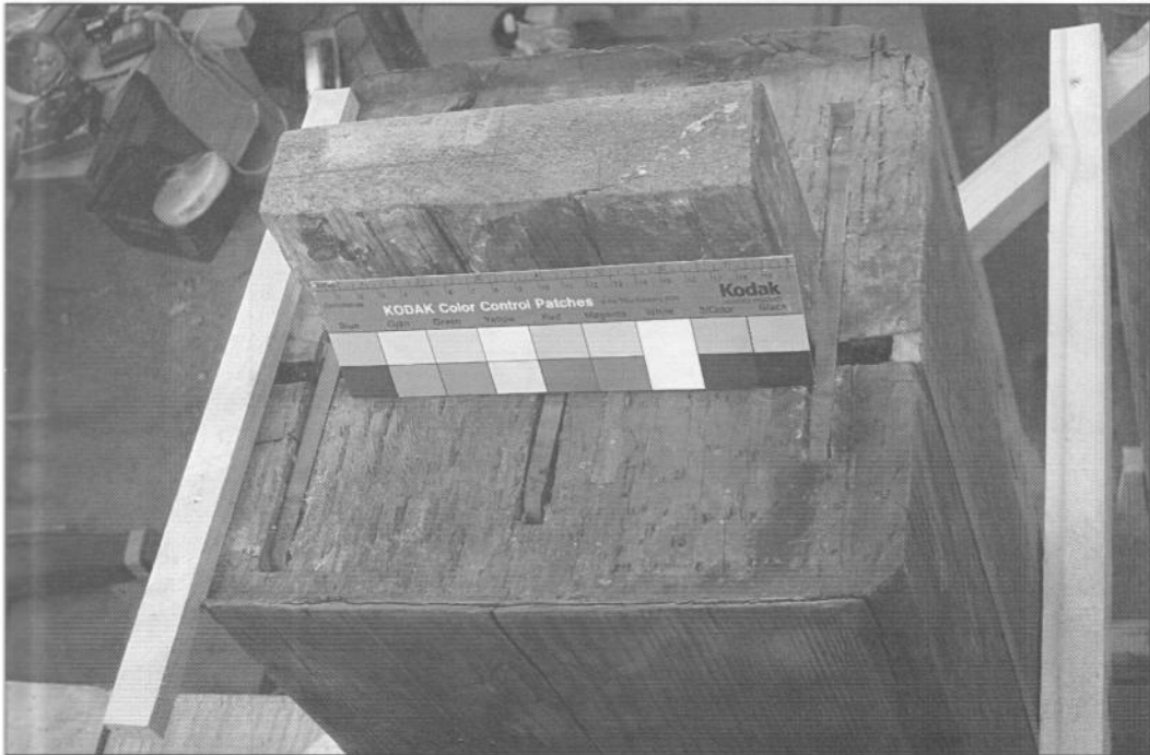
Strengthening Wooden Pillar During Conservation, Kyouto, Japan
