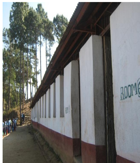
School Building of Sharada Secondary School Gelu, Ramechhap
