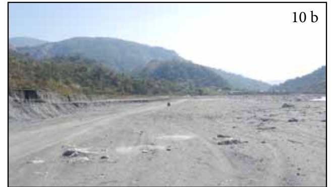
Fig. 10: Field photograph of the landslides at upper reaches of Dahare Khola (10a) and its impact to the road alignment at the downstream, around Ullikhola village (10b).
