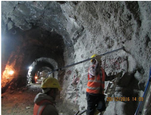
Installation of Rock Bolts
