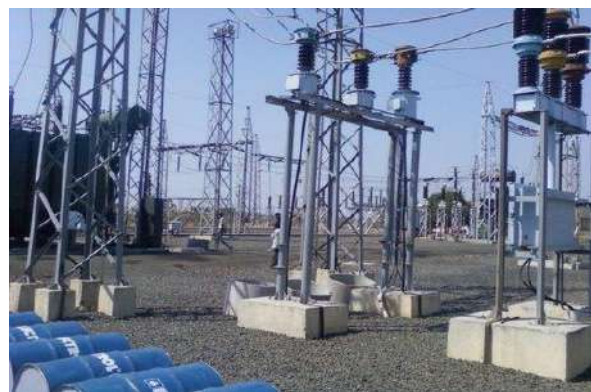
Civil-Structures Supporting Electrical Components
