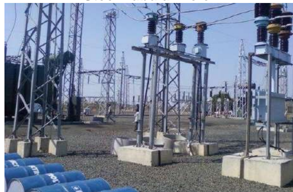
Civil-Structures Supporting Electrical Components
