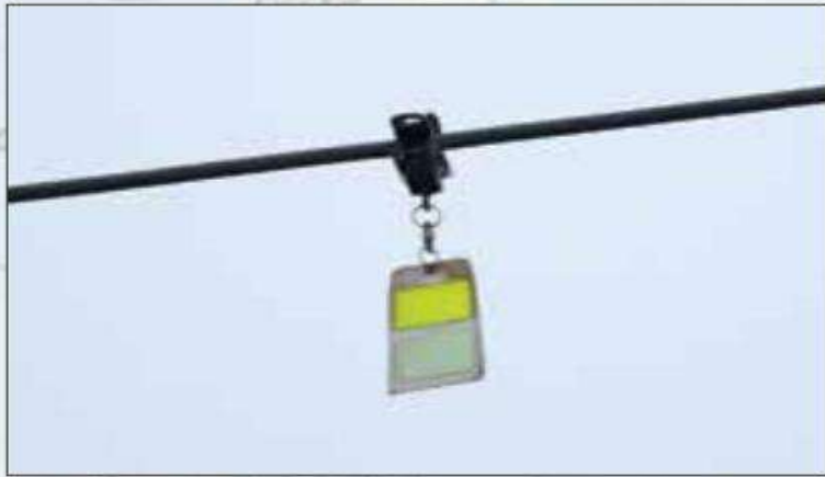
Bird Diverting Reflector
