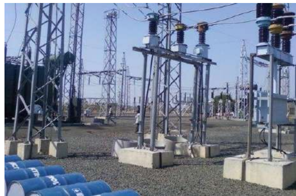
Civil-Structures Supporting Electrical Components
