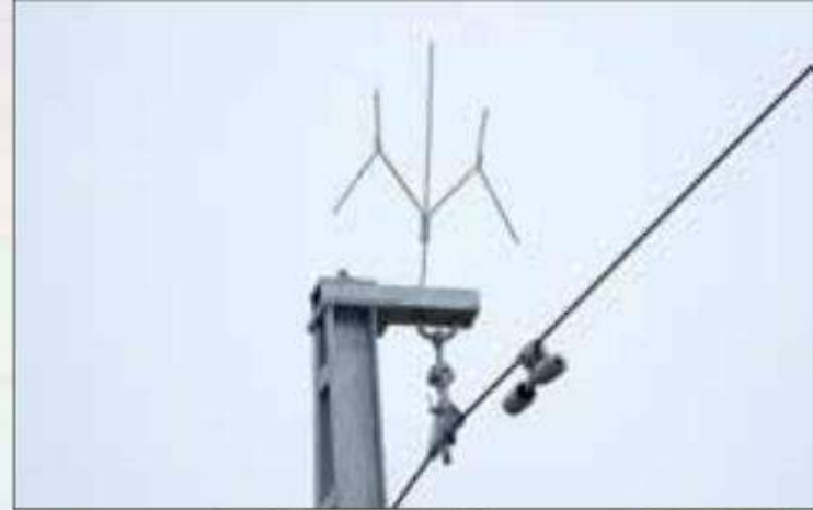
Wishbone Prevents Bird Landing on Wire
