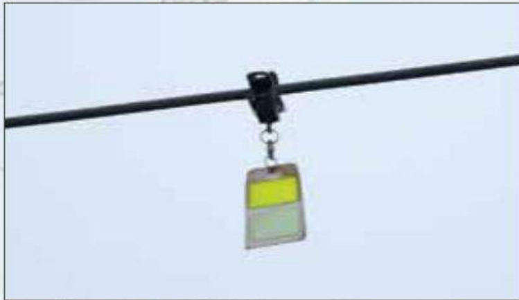
Bird Diverting Reflector
