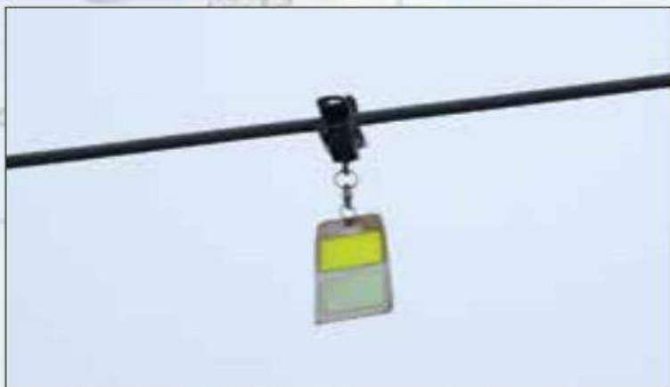
Bird Diverting Reflector
