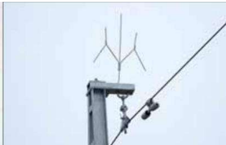
Wishbone Prevents Bird Landing on Wire
