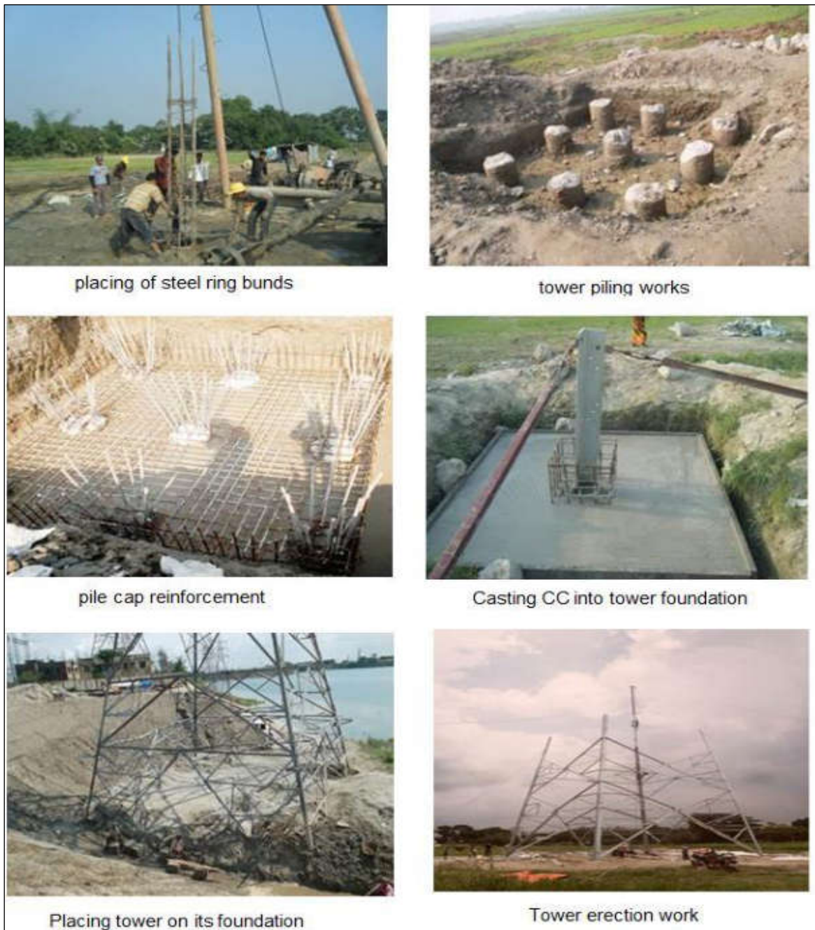
FIGURE 22: TYPICAL CIVIL WORKS FOR INSTALLATION OF TRANSMISSION LINE
