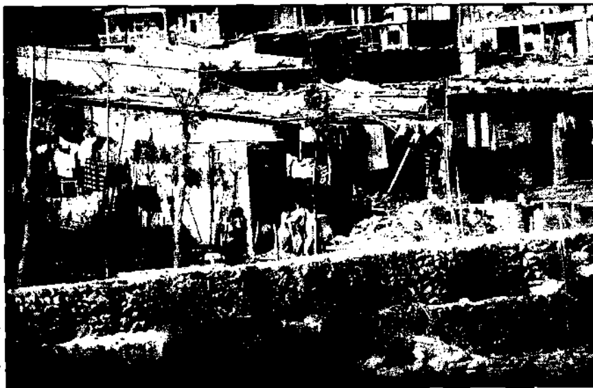
Temporary Flood Protection along Squatter Settlement
