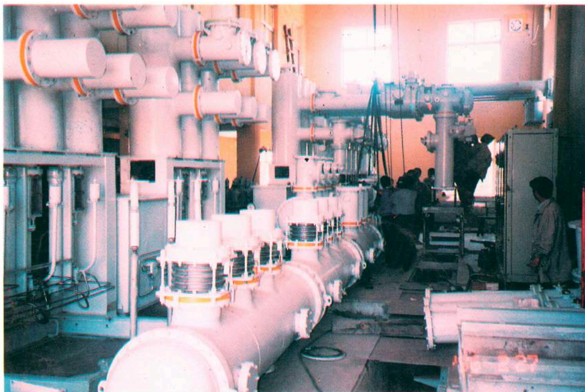
Installation work of 66 KV GIS in Teku Substation
