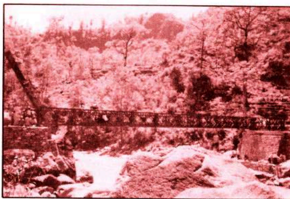
Bailley Bridge Construction
