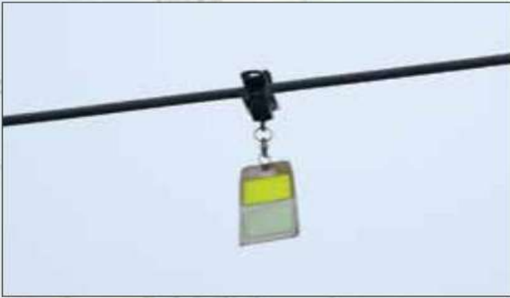
Bird Diverting Reflector
