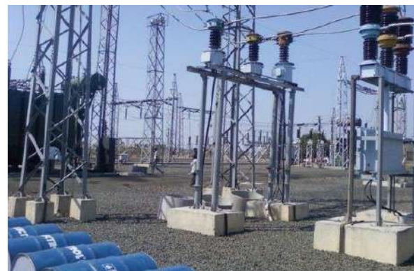
Civil-Structures Supporting Electrical Components
