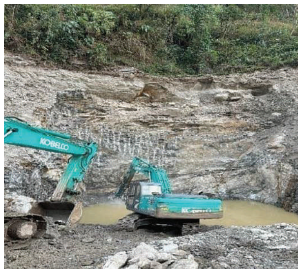
Bridge foundation excavation at Chhongryak
