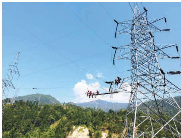
Conductor stringing at New Khimti Substation
