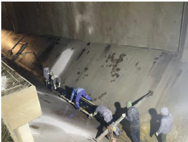
Replacement of Eroded plates of Desander Basin
