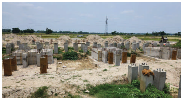
Equipment Foundation Works at Keraun 132/33kV Substation
