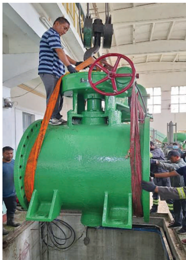
Reinstallation of MIV during overhauling of unit no. 1
