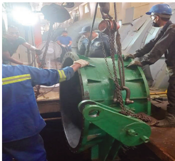
Reinstallation of MIV for unit No.7
