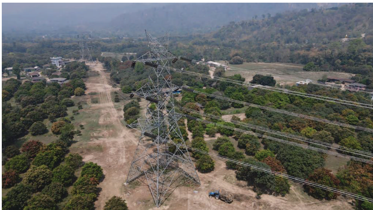
QUAD ACSR Moose Conductor Stringing
