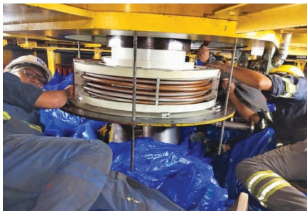
Repair of eroded upper guide bearing oil cooler
