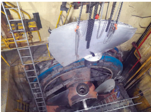
Dismantling and Lifting of Runner Blade
