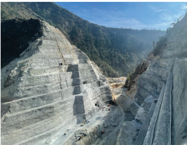
Dam Slope Excavation and support works
