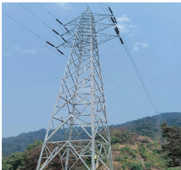
Narrow Based Tower no.54 after the completion at Daunne Danda
