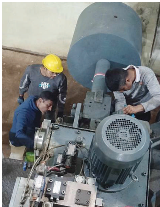
Repair and maintenance of Main Inlet Valve servomotor
