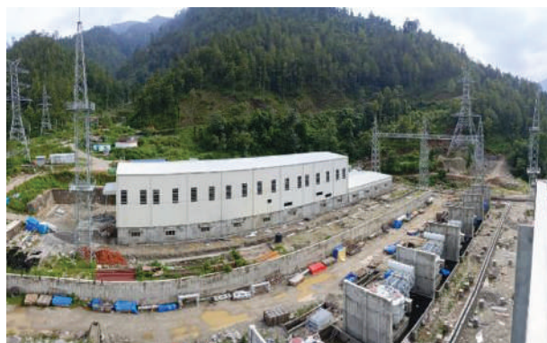
400kV GIS Building and Transformer Banks
