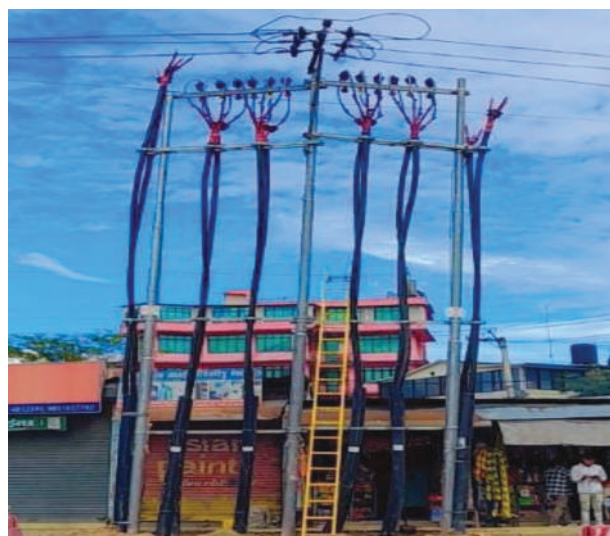
Overhead termination of Underground Cables
