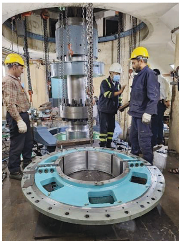
Guide Bearing Repair/Replacement work
