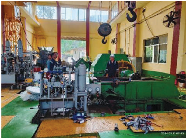
Turbine Overhauling Works of Unit #01
