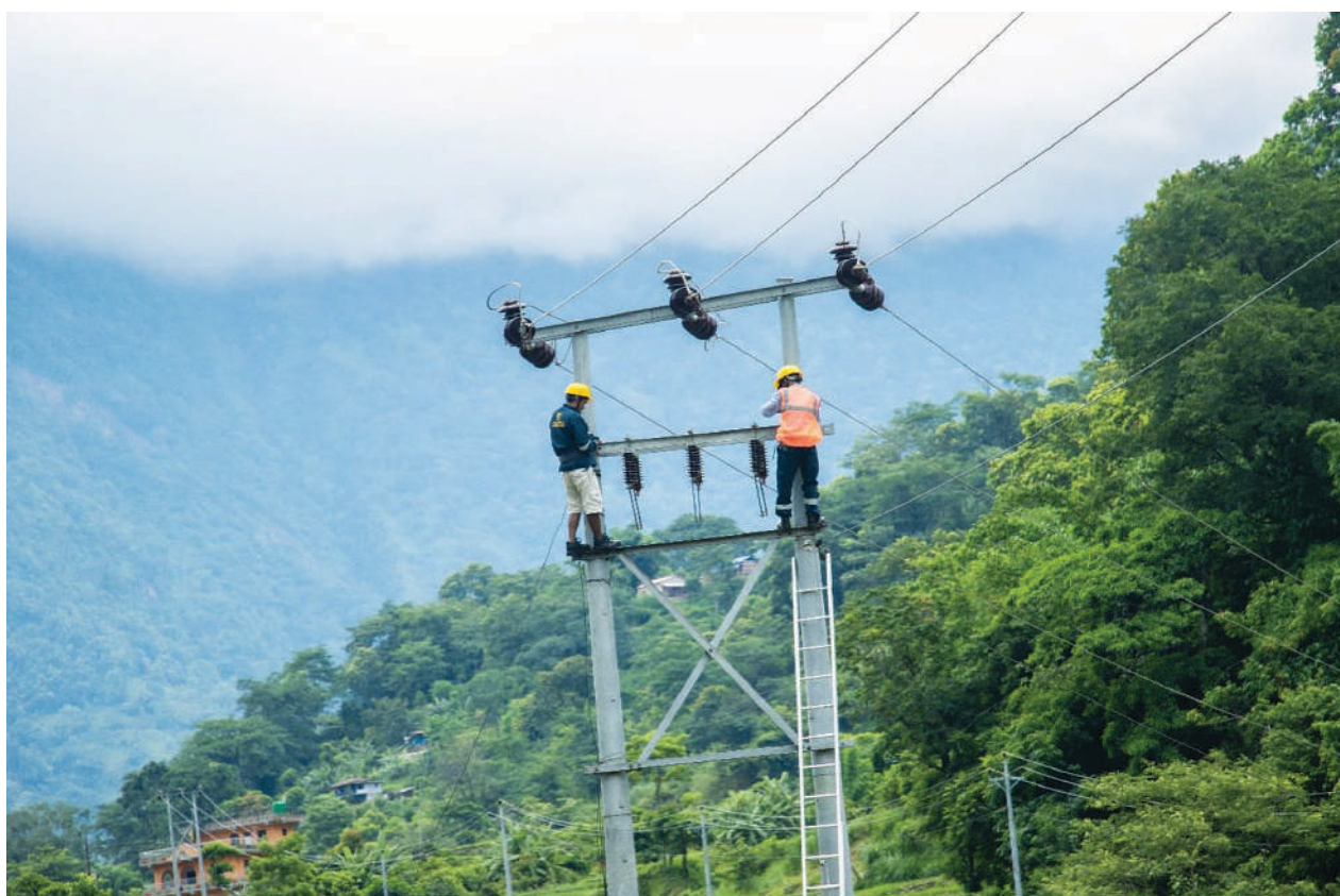
33 kV Line construction works by Lamjung Distribution Center
