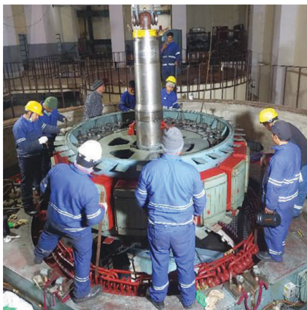
Installation of Rotor Pole after repair of rotor pole connector of Unit No. 2
