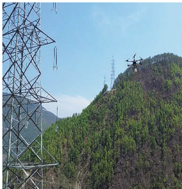
Stringing work by using drone
