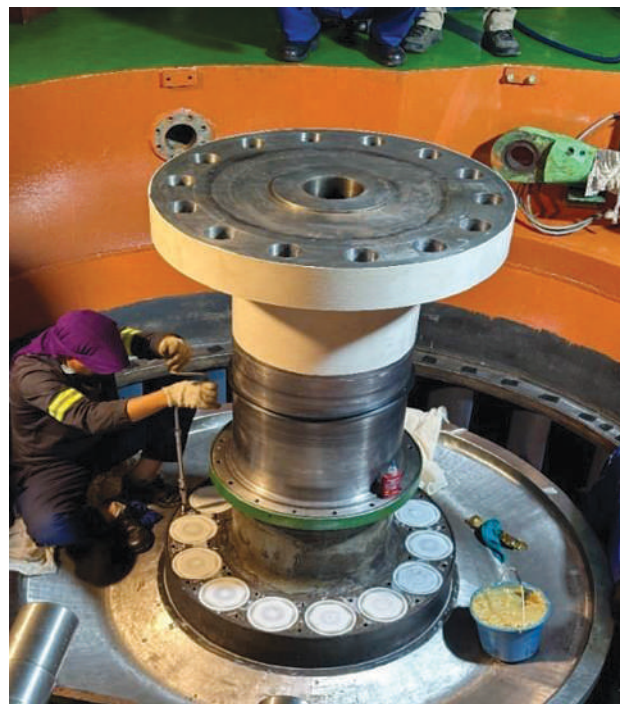
After assembly photo of runner shaft and runner during overhauling of Unit No-1
