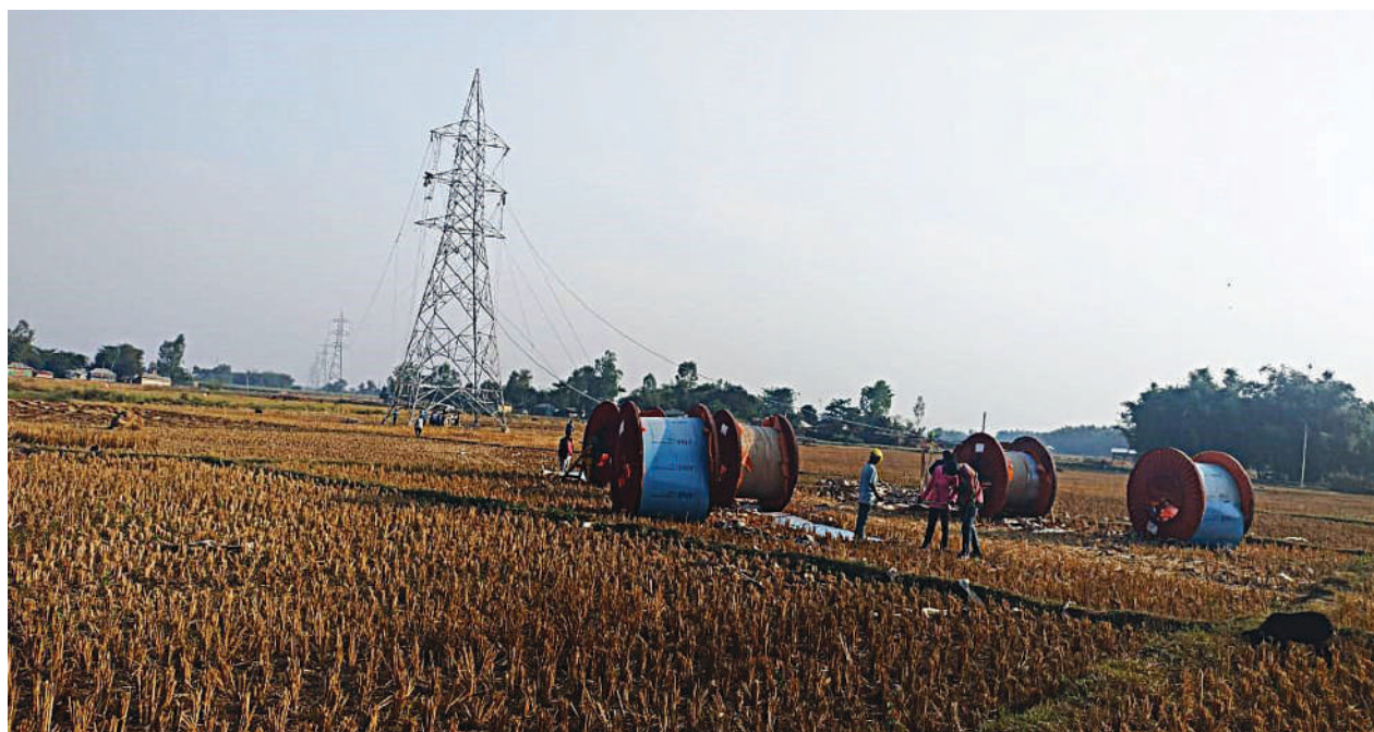
Conductor Stringing Works on going
