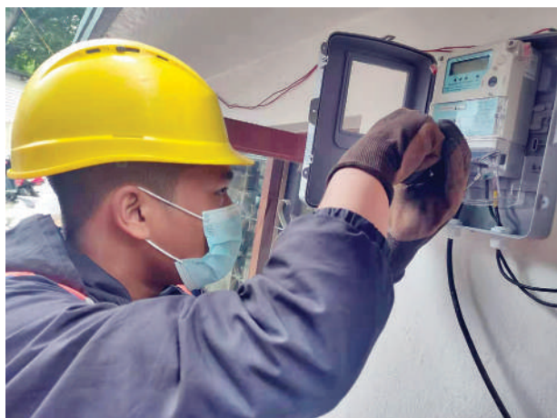
Installation of Smart Meter at Residential Consumer
