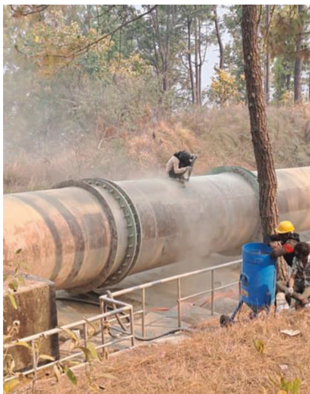
Sand blasting for surface preparation at Penstock Pipeline
