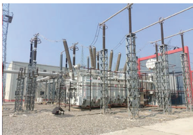
315 MVA Transformers at Inaruwa substation
