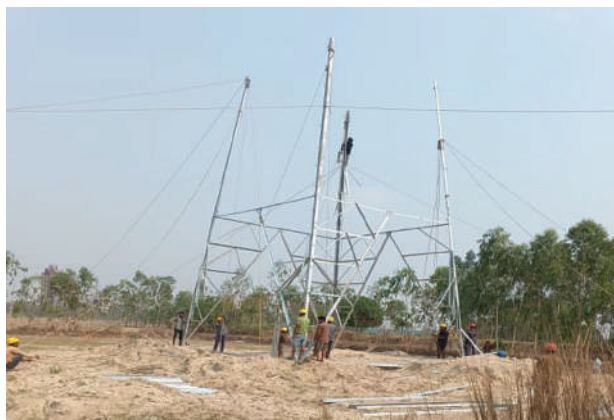
Tower Erection works ongoing
