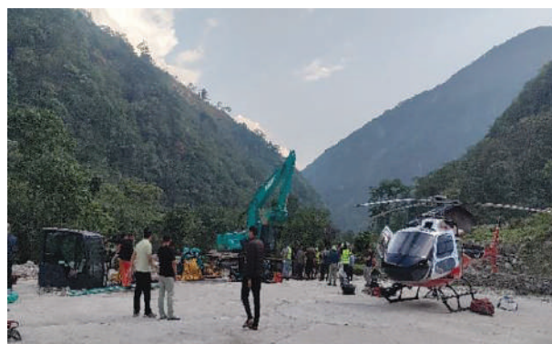
Heli lifting of construction equipment for access road construction
