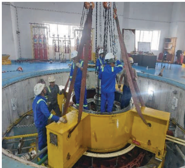
Overhauling of Unit No.1
