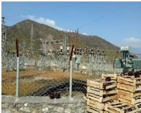
Figure 3-2: Tapping Point of DL at Bay extension point at kudu substation
