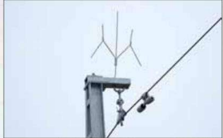
Wishbone Prevents Bird Landing on Wire
