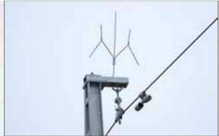
Wishbone Prevents Bird Landing on Wire
