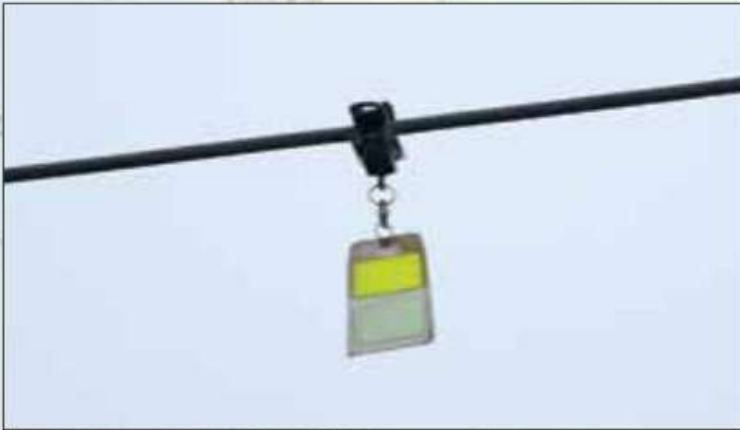
Bird Diverting Reflector
