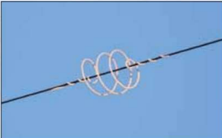
White Spiral in Wire Improves Visibility of Wire
