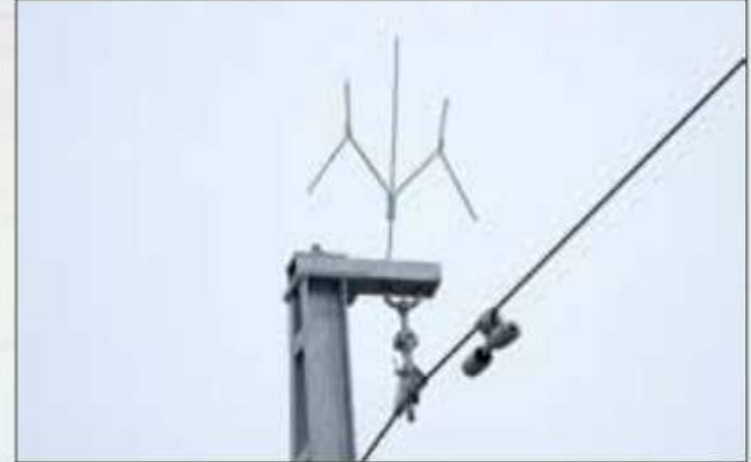
Wishbone Prevents Birds Landing on Wire
