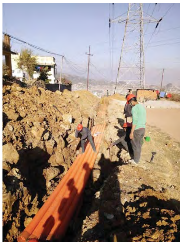
Under construction under ground cable laying work
