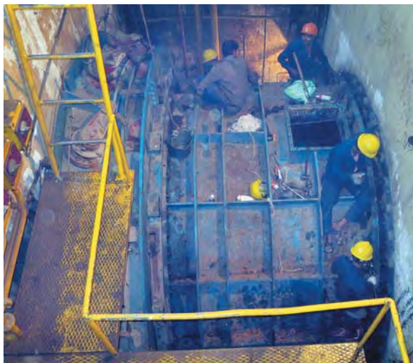
Unit No. 3 Turbine Cover Opening.
