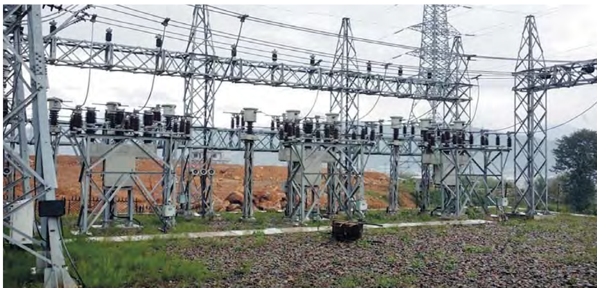
33 kV Bay extension work at Matatirtha Substation
