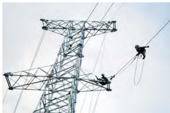
Conductor stringing work of Bhulbhule to Middle Marsyangdi 132kV T/L Project
