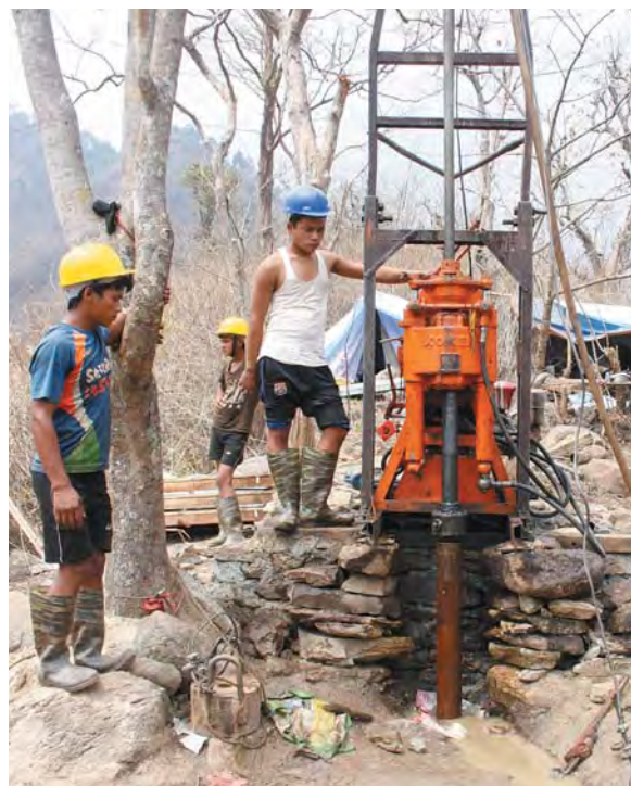
Core Drilling Work at Dam Site
