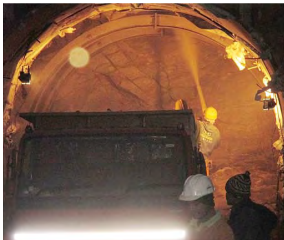
Application of Shotcrete in Test Adit Tunnel
