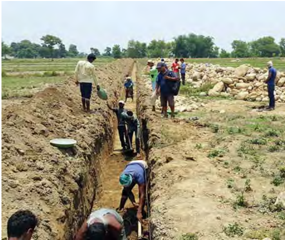
Compound Wall Foundation of Mainahiya Substation
