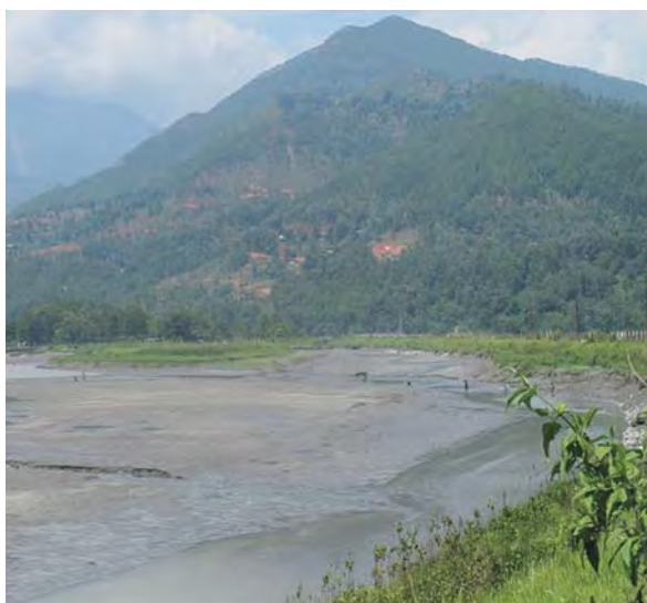
Sediment Deposition in the Reservoir observed during emptying
