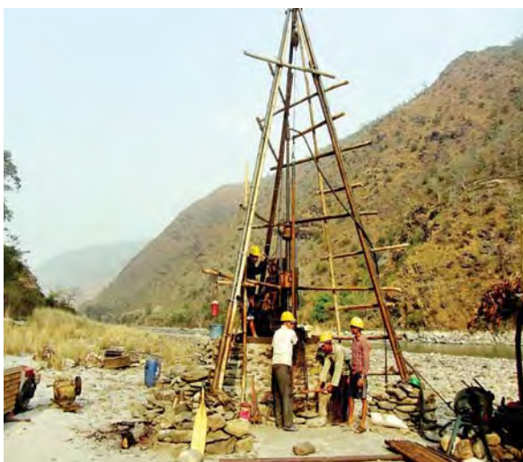
Core drilling at Dam site of Tamor Storage Hydroelectric Project.
