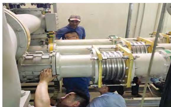
Installation of GIS at Marsyangdi Power Plant Switchyard
