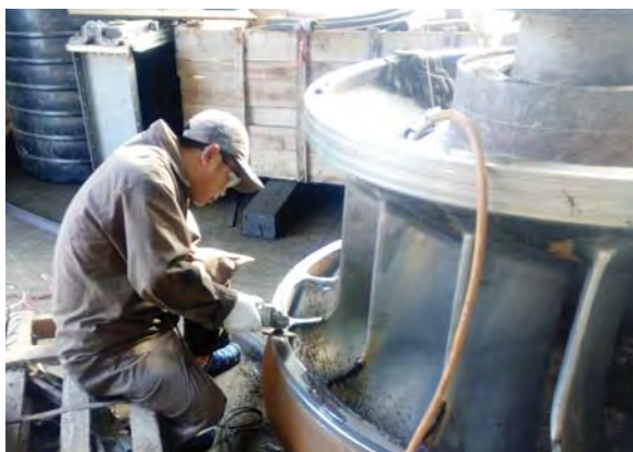
Repairing of runner during overhauling of unit no. 2
