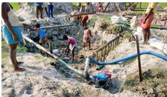
Pit Excavation work for Tower Foundation
