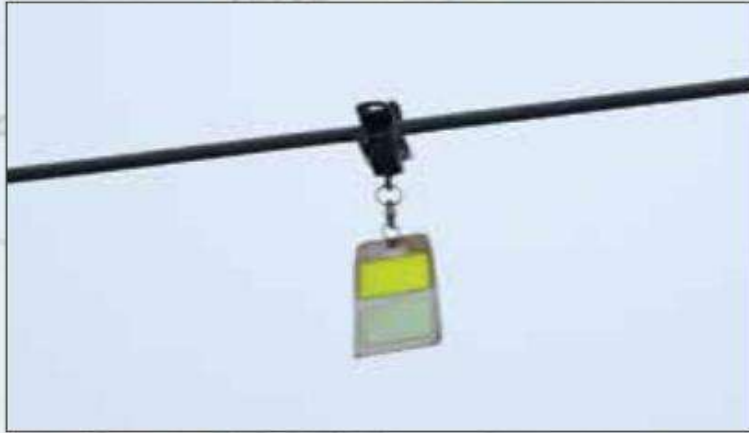
Bird Diverting Reflector
