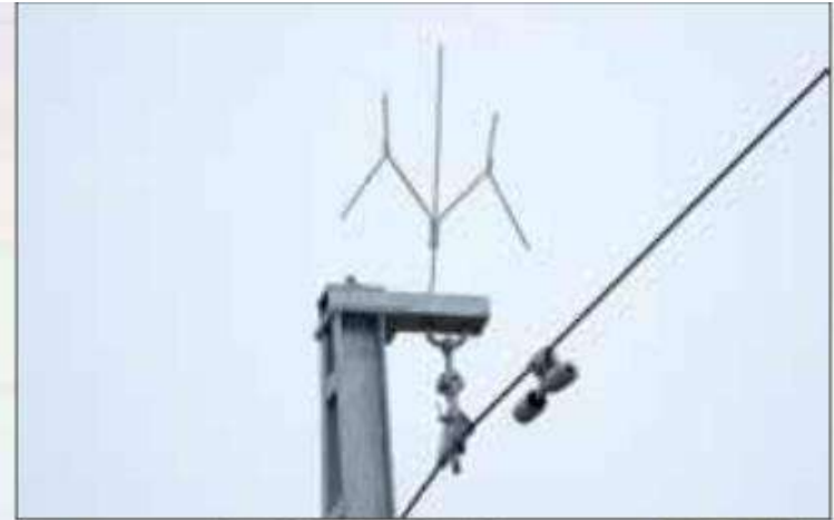
Wishbone Prevents Bird Landing on Wire
