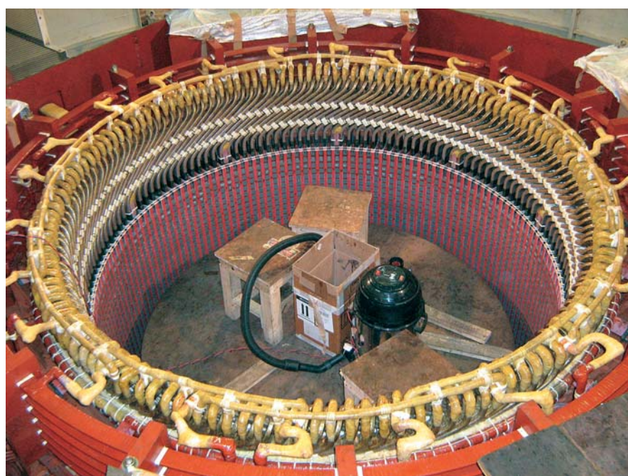
Repaired Stator of Generator No. 2 of Kulekhani-II HPS
