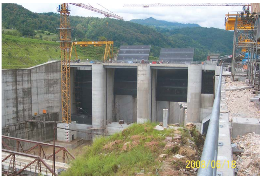
Installation of Radial Gates at Headworks (View from Upstream)
