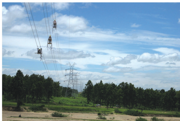
Khimti-Dhalkebar 220kV Transmission Line Conductor Stringing Work
