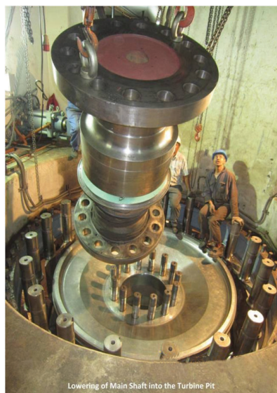
Lowering of Main Shaft into the Turbine Pit
