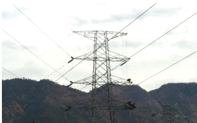
Live Line 2 nd Circuit Stringing work is in progress
