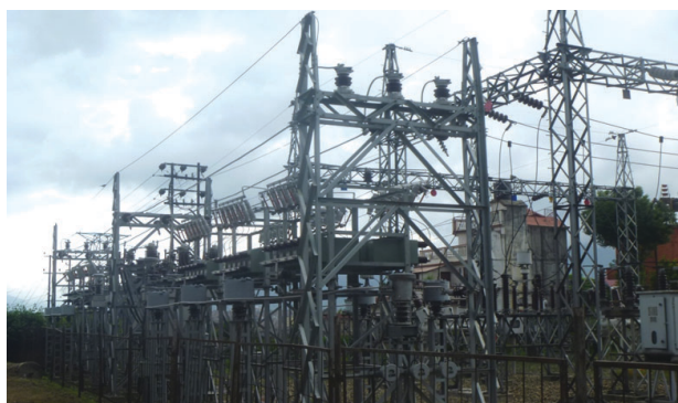
Newly Installed Capacitor Bank at 66/11kV Baneshwor Grid Substation
