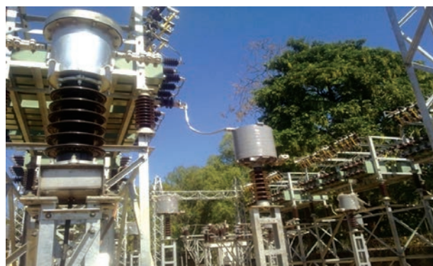
Capacitor Bank Installed at Butwal Substation
