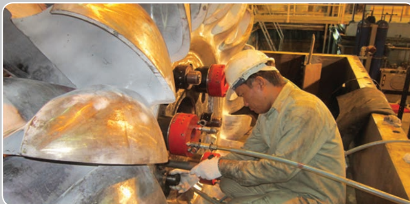
Figure: Fitting of Repaired Pelton Runner on Unit-2 in Progress
