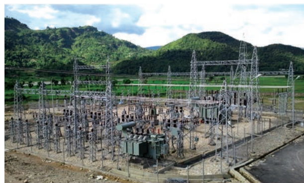
Shyangja 132/33kV, 30MVA Substation under construction
