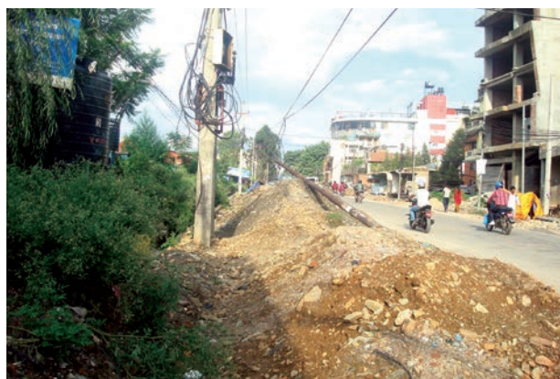
Dismantling and realignment of pole
