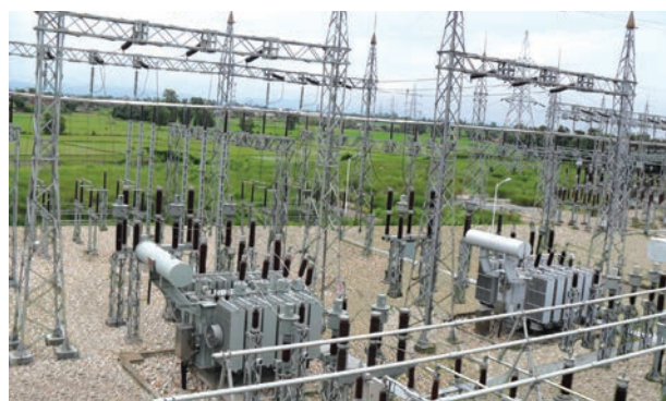
Power Transformer at New Parwanipur S/S
