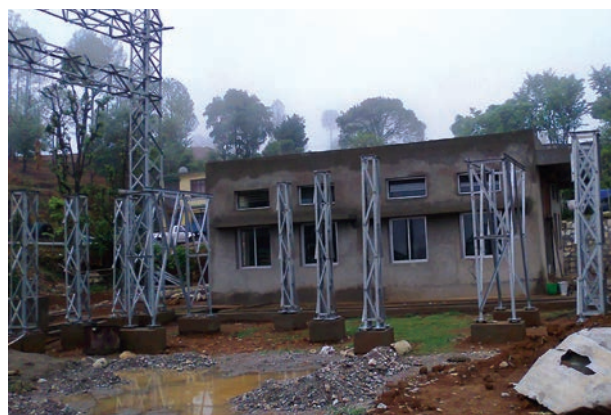
33-11 KV Substation at Dailekh under construction
