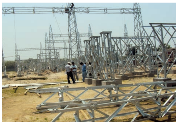
132/33kV, 30MVA Damak Substation under construction
