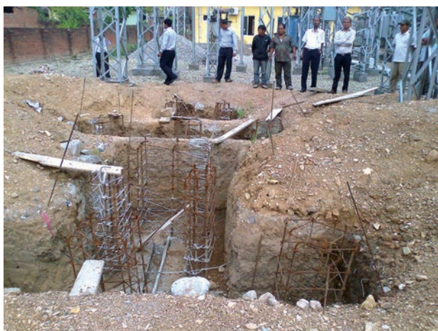
33KV Bay at Ghorahi under construction
