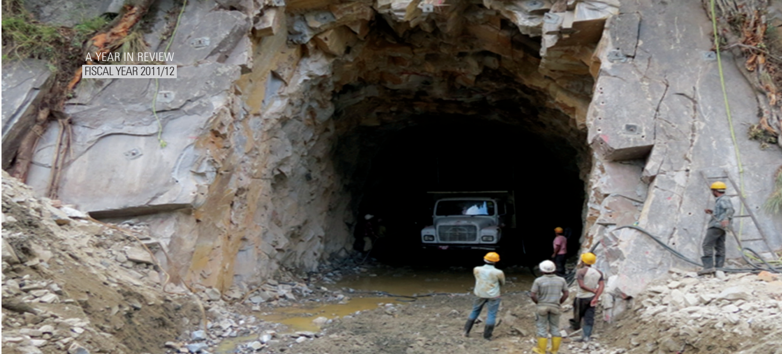
Figure 1: Construction of Test Adit Tunnel
