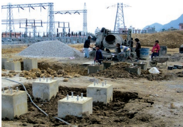
132kV Equipment Foundation Work at Matatirtha Substation
