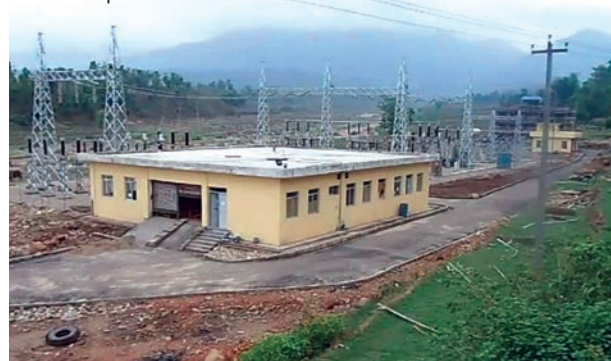
Hapure 132/33kV, 30MVA Substation under Construction
