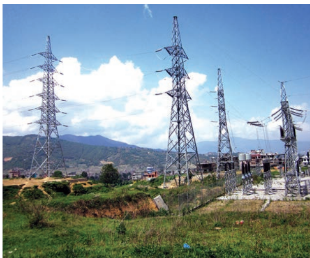
4 Circuit Tower at Matatirtha Substation for Loop in Loop Out Connection from Siuchatar
