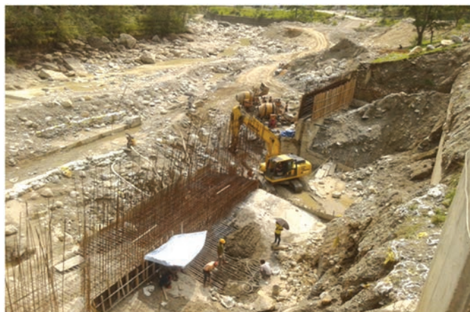
RCC Works of Retaining Structure on Downstream of Undersluice Gate of Modi Khola
