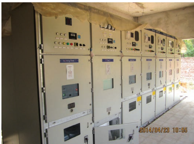
12 kV Indoor switchgears installed at Barhathawa substation in Sarlahi district
