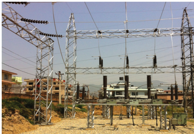
New 132kV Bay Expansion for 2 nd Circuit connection at Siuchatar Substation
