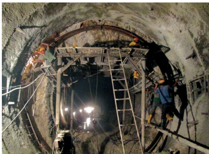
Photo: Tunnel squeezing treatment work in Chameliya HEP
