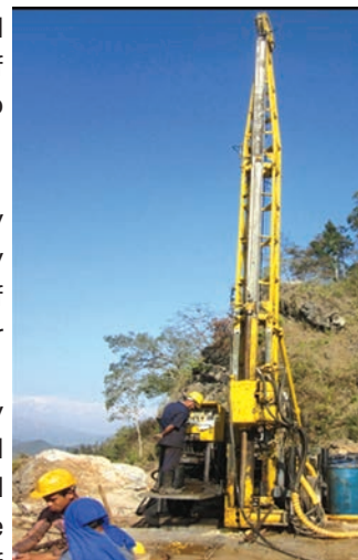
Core drilling at Dam site of Tanahu Hydropower Project.
