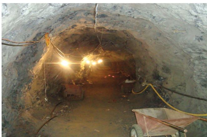
Test audit excavation for additional geological study at dam site.
