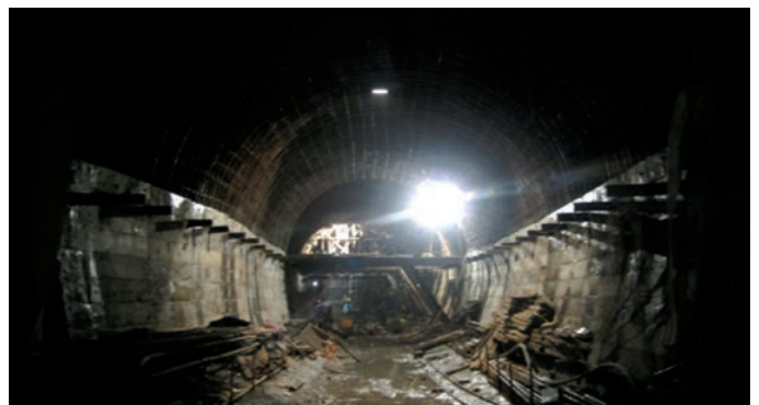
Concrete lining works in Forebay of Kulekhani III HEP
