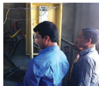
Photo 2: Data being downloaded from TOD meter during field visit to the consumers under Tikapur DCS.
