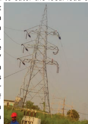
Butwal-Kohalpur 2 nd Circuit Stringing Work is in Progress
