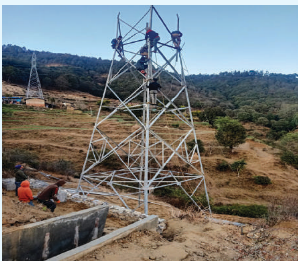
132 kV Lattice Tower Construction at Syaule Substation
