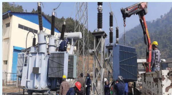
Replacement of Power Transformer Radiator
