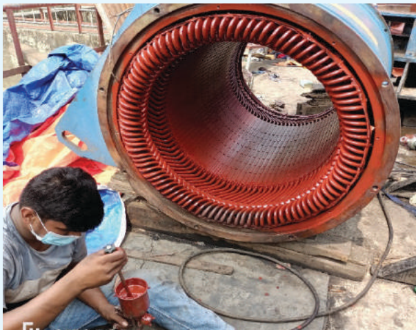
Generator Stator
