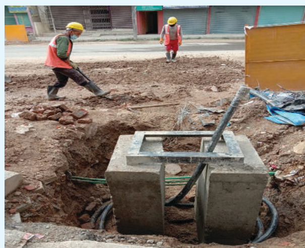
Cable Looping around E1 Panel at Chabahil Site
