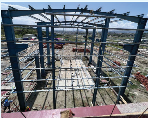
PEB erection of GIS Hall- Changunarayan Substation
