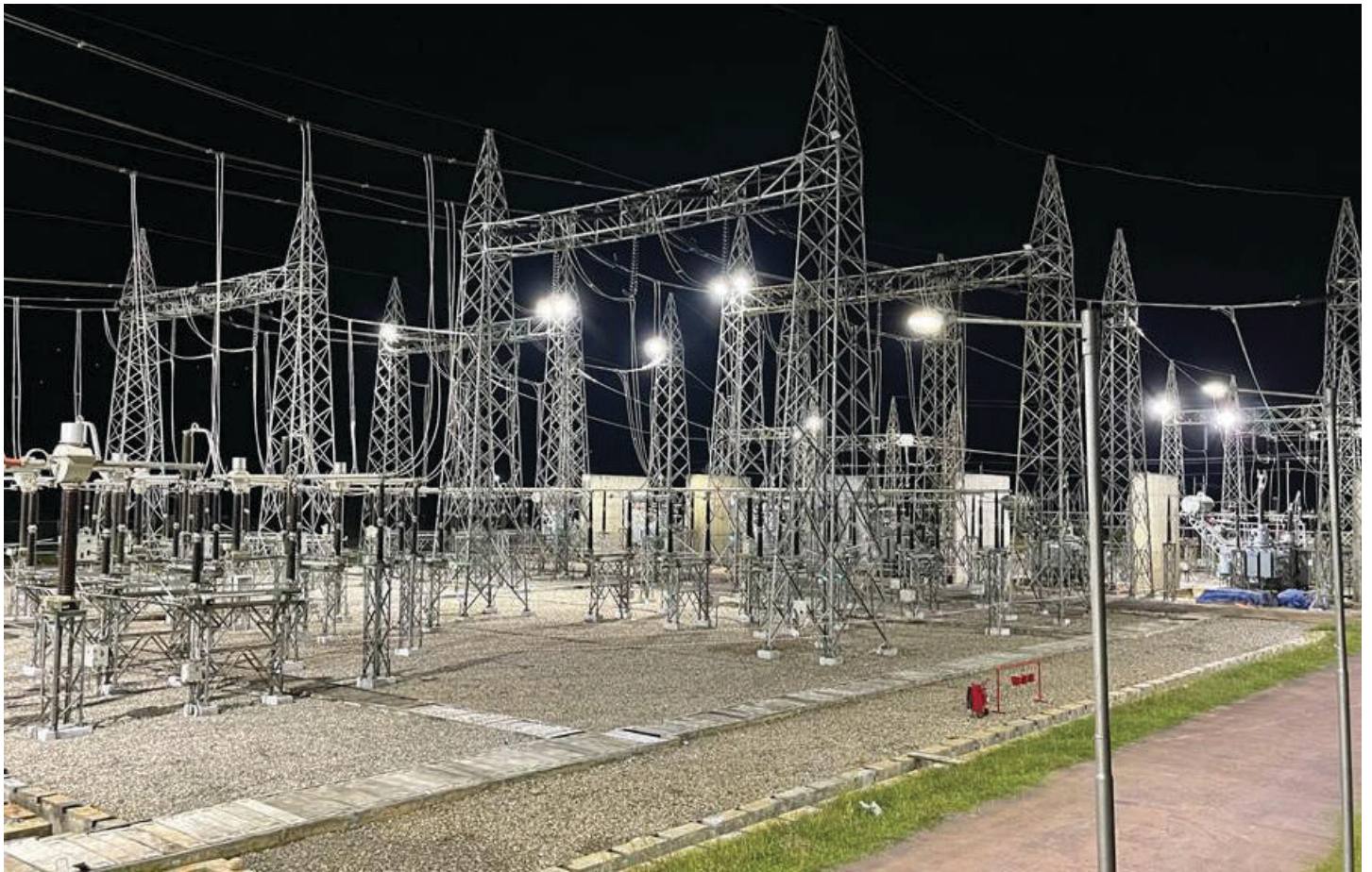
Tumlingtar 220/132 kV (200 MVA) Substation
