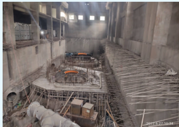
SHEP Headwork and Machine Installation Work in Powerhouse
