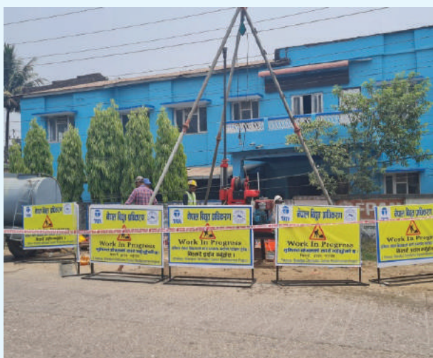
Soil Investigation Work Using Rotary Drilling Machine
