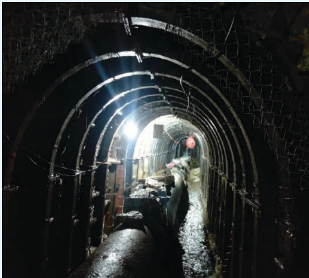
Protection Works of Tunnel at Sundarijal HPS
