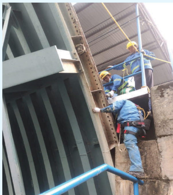
Repair and Maintenance of Spillway Radial Gate
