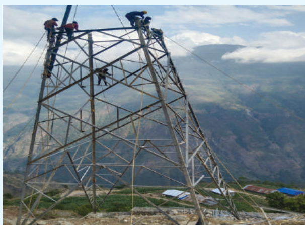
Tower Erection Works
