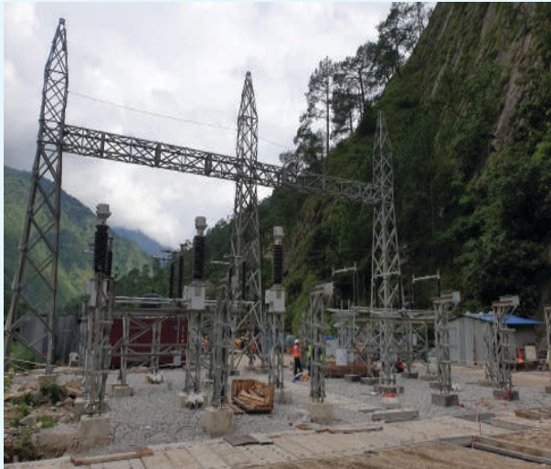
Take- Off Yard Construction in Progress
