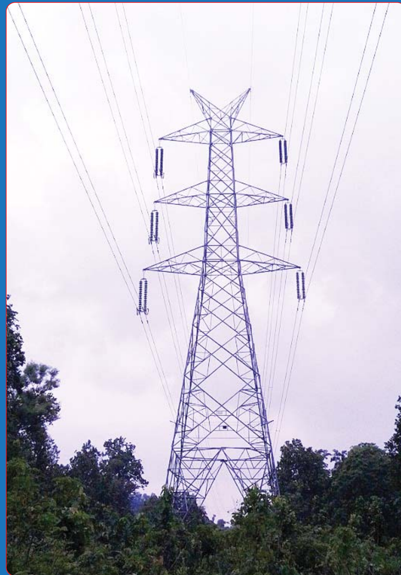
Khimti - Dhalkebar 220 KV Tower
