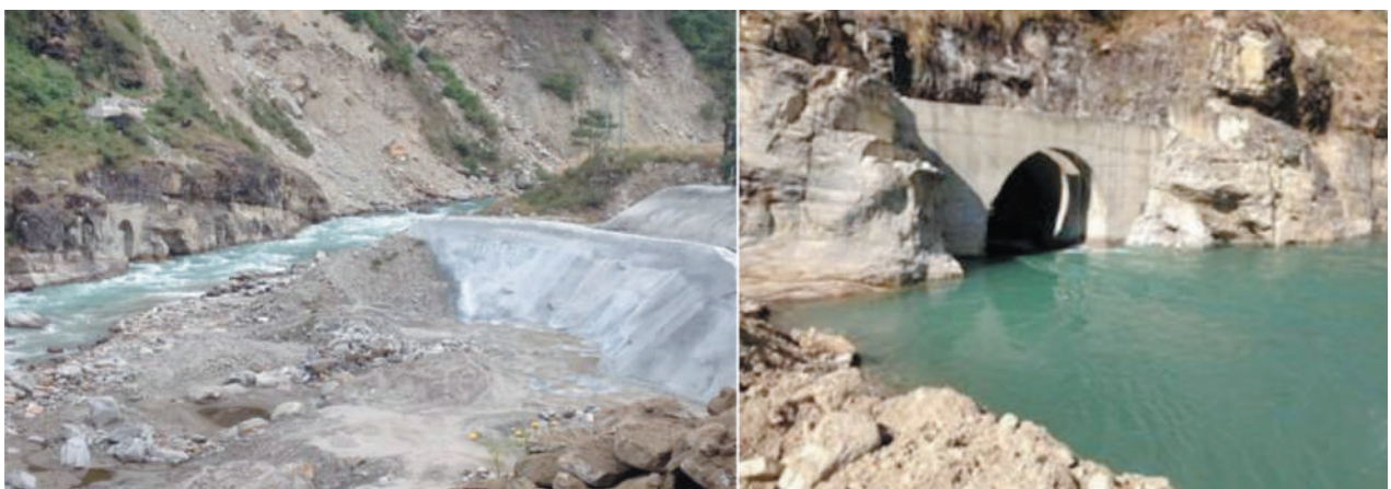
River diversion of Middle Bhotekoshi HEP before and after diversion
