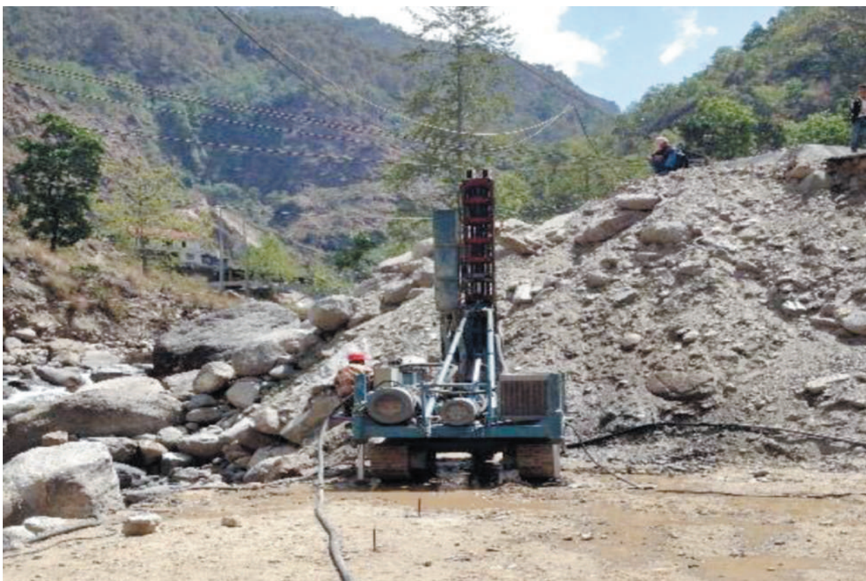
Jet grouting at the Cofferdam of Madhya Bhotekoshi HEP
