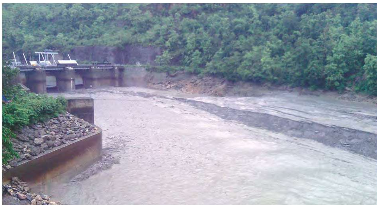
Flushing of Reservoir during Monsoon
