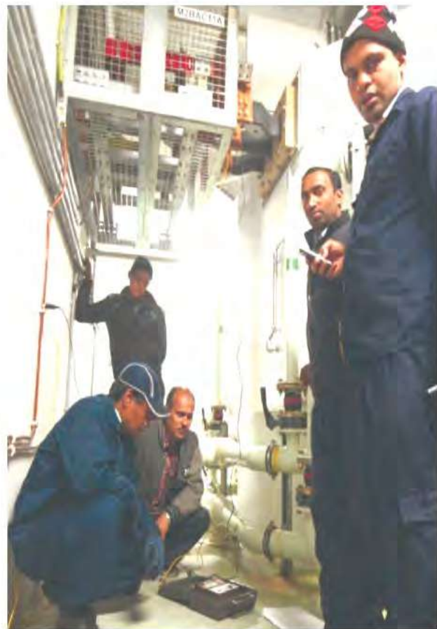
Meggering of Generator Stator in Unit No. 1
