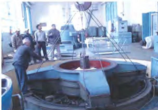
Dismantling of Upper Bracket During Overhauling
