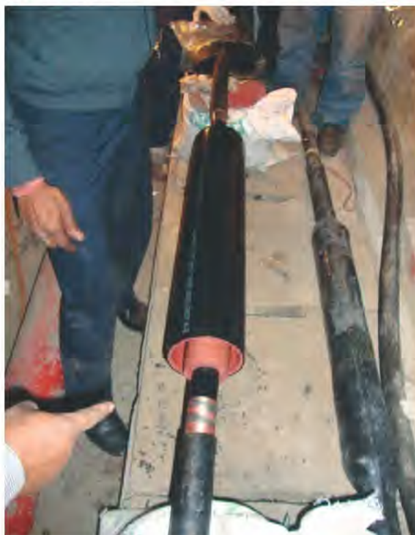
66 kV Heat Shrinkable Straight Through Jointing in Progress
