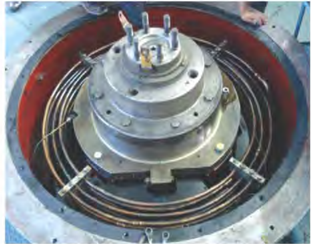
Dismantling of Upper Guide and Thrust Bearing
