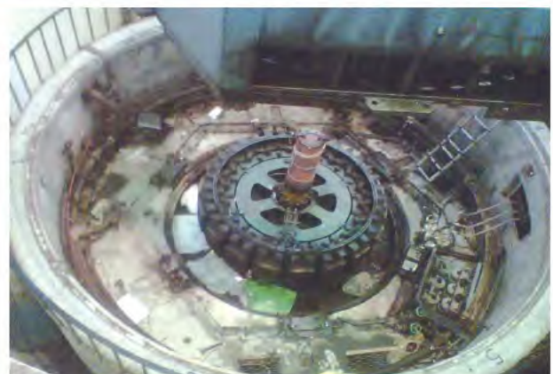
Generator during Overhauling
