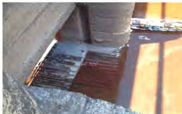
Erosion of Seal Beam in Gate
