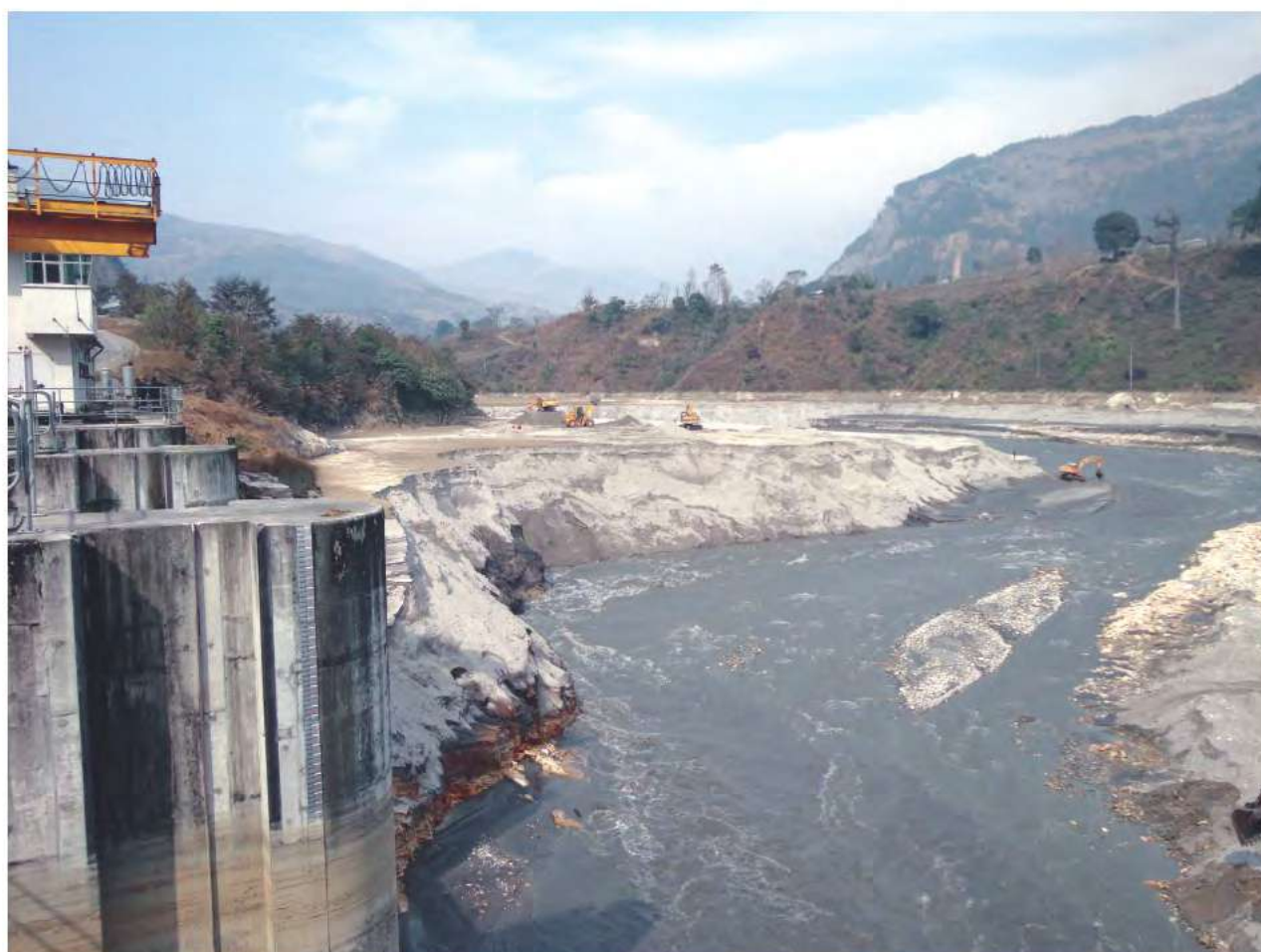
Reservoir Flushing and Sanbd Removal during Repair Work Carried Out in February 2012 in Middle Marsyangdi Hydropower Station
