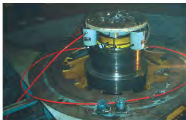
Hydraulic Jacking to Uplift Thrust Collar
