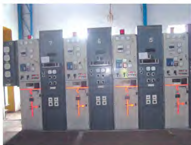
Recently Installed VCB with Control and Relay Panel
