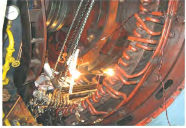
Replacement of Stator
