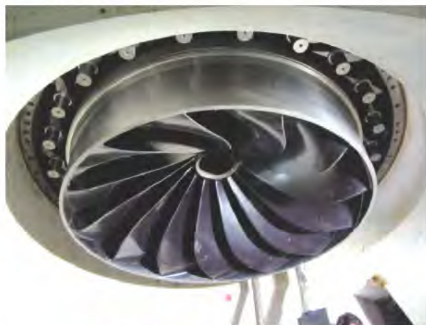
New Runner after Installed in Unit No. 1
