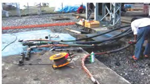
Repair of 6.6 kV Power Cable of Transformer.
