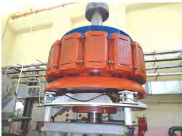
Draw Out of Rotor of Unit No. 1 during Overhauling
