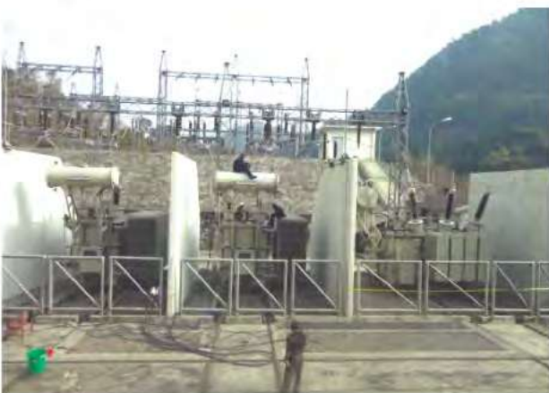
Oil Filtration of 14.5 MVA Power Transformers
