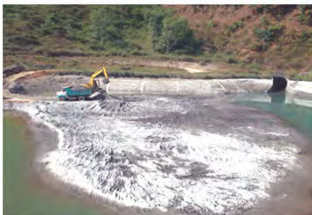
Removal of Sand from Forebay
