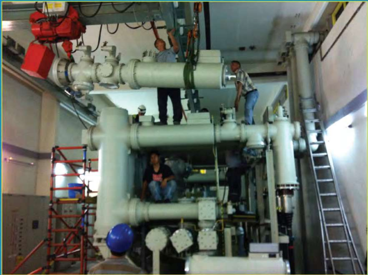
Replacement Works of GIS CT in Marsyangdi Hydropower Station
