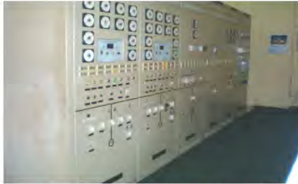
Circuit Breakers with Control and Relay Panel
