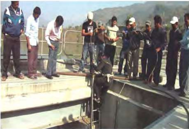
Divers (Gotakhor) for Checking Underwater Obstacles at Spillway Gate No. 1.
