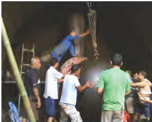
Turbine Hub Dismantling
