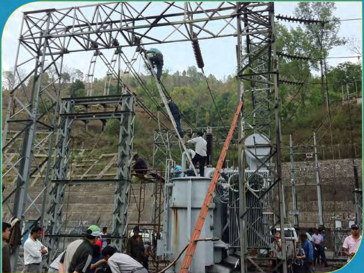
Replacement of Single Phase 132 KV Power Transformer, 'B' Phase by Spare Transformer in Kulekhani-II Hydropower Station
