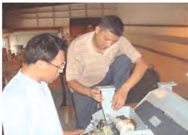
UHF PD Measurement of Line and Unit Bay
