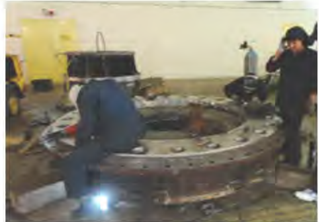
Maintenance Works in Bottom Ring
