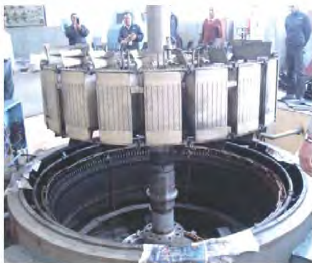
Generator Rotor During Overhauling
