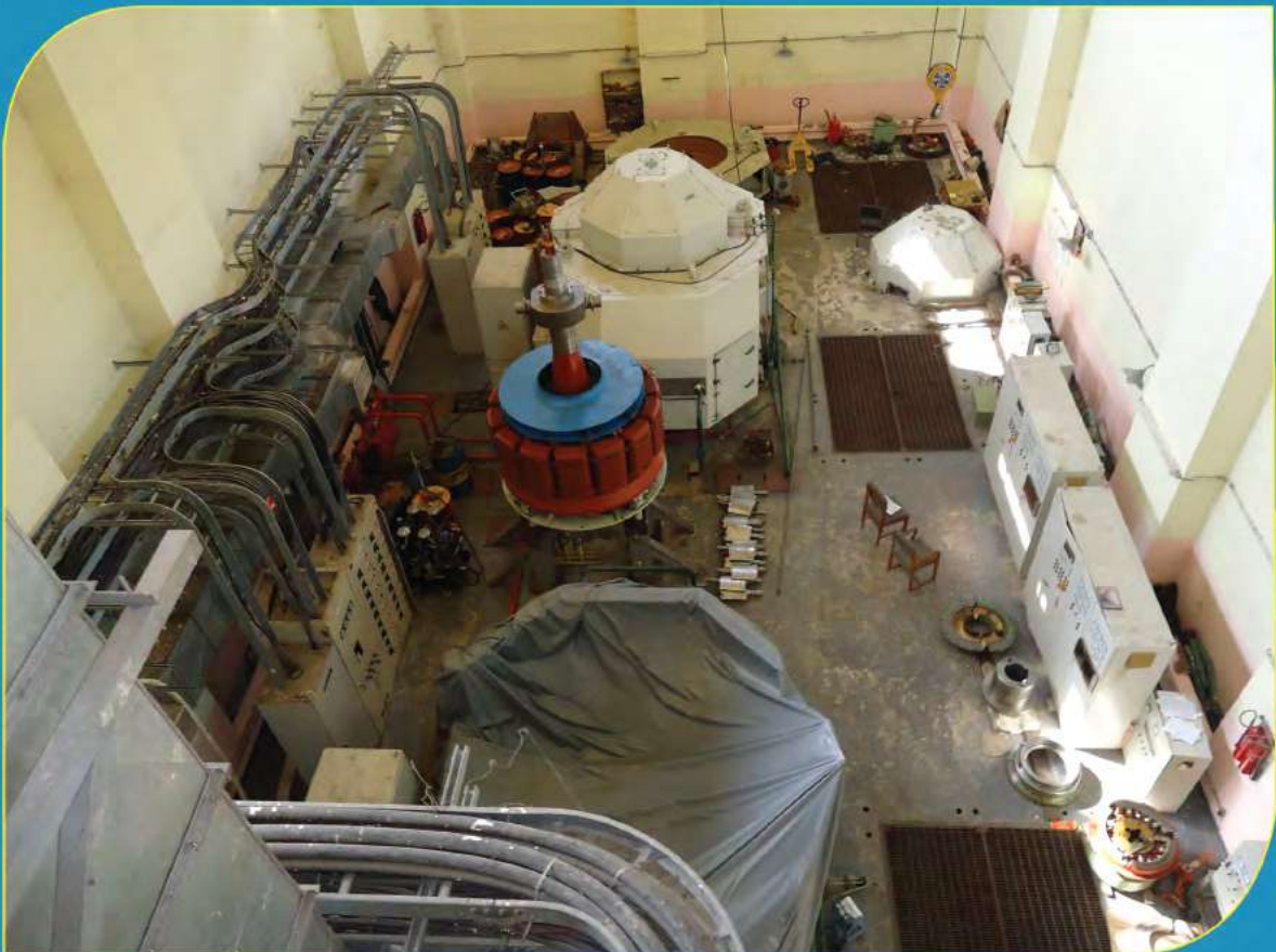
Overhauling of Unit No. 1 of Modi Hydropower Station
