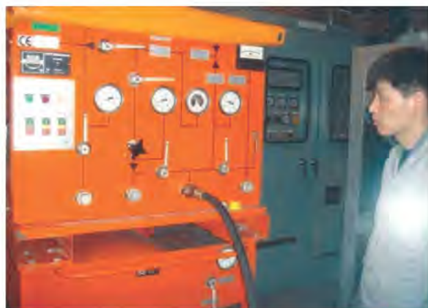
Removal, Evacuation and Refilling of SF 6 Gas in Butwal #1 Line Bay PT.
