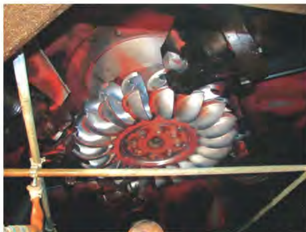
Inspection of Pelton Runner
