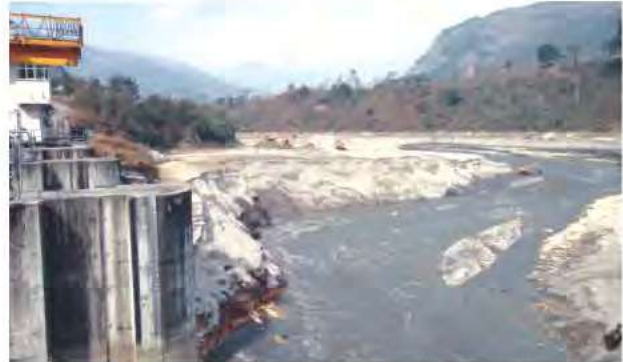
Removal of Reservoir Accumulated Sand
