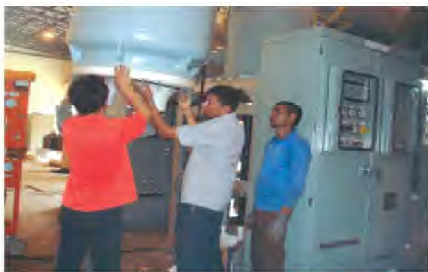
Installation of New PT at Unit # 1 Transformer Bay.
