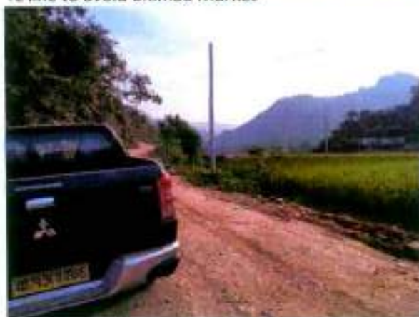
Pole crossing the road
