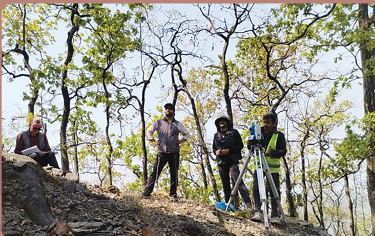
Engineering survey on temporary access tracks required for the construction of tower pads along the route of the transmission line being conducted.
