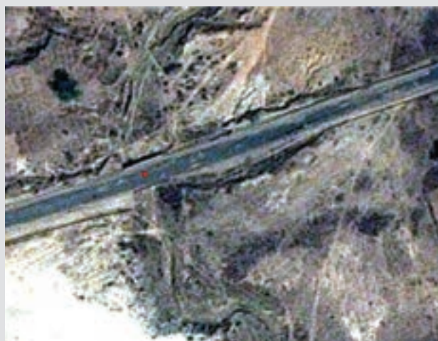
Photo B5.2: Example of Bridge Identification
