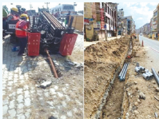
HDD & Pipe Laying Work in Process
