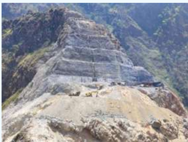
Excavation of Dam Abutment (Right Bank)
