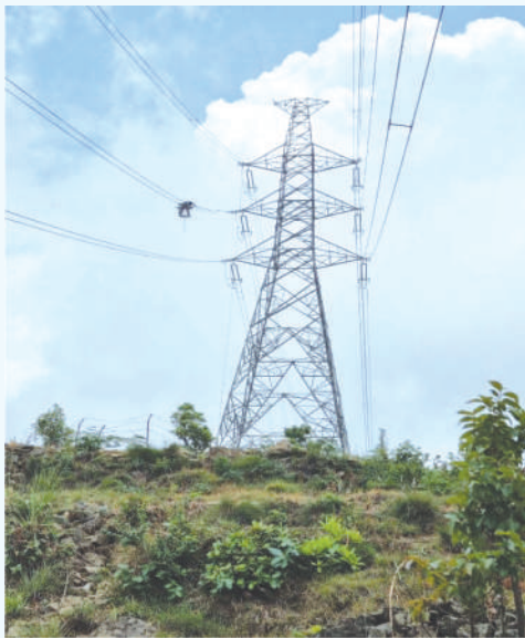
Conductor Stringing Works
