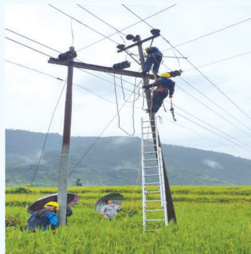
11 kV HT Line Maintenance under Pyuthan DC
