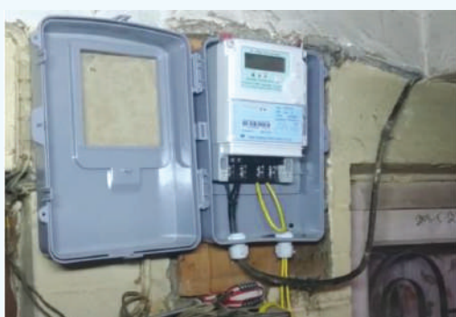
Smart Meter Installation
