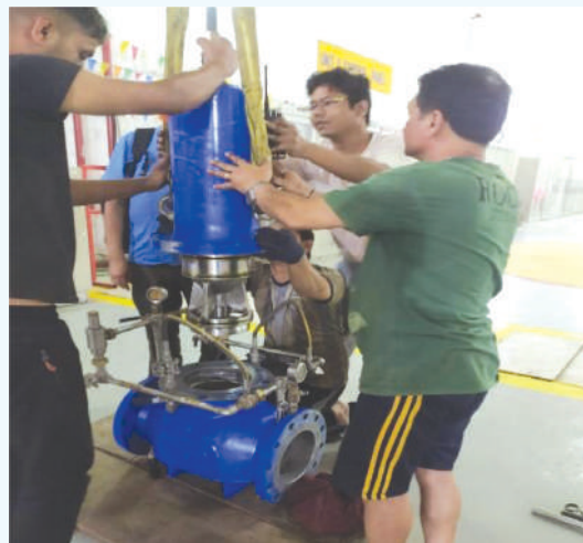
Assembly & Fitting of Repaired Pressure Reducing Valve of Unit-2
