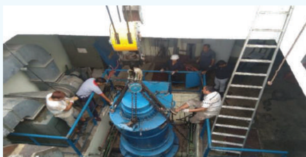
Generator Dismantling for Stator Repair
