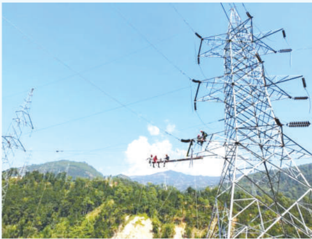
Conductor Restringing Works at New Khimti Substation
