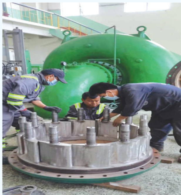
Guide Vane Assembly Works
