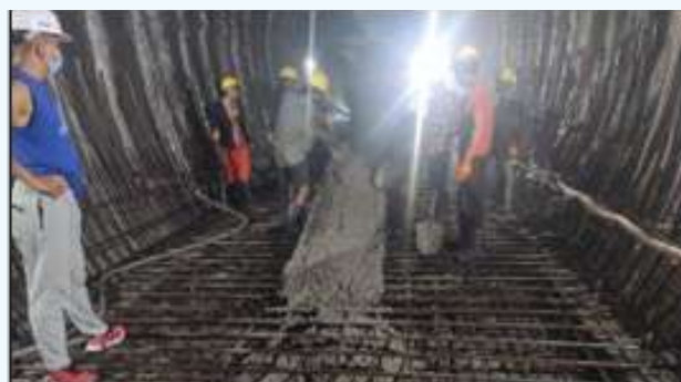
HRT Invert Concreting
