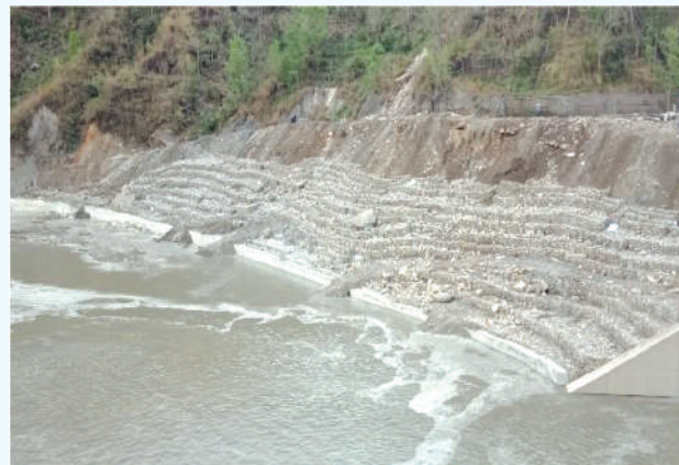
Left Bank Protection Works
