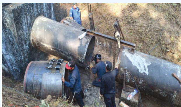
Penstock Rectification Work
