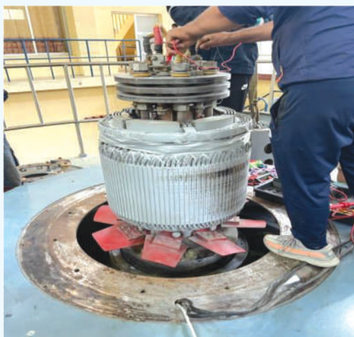
Repairing of Excitation System.
