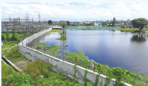
RCC Boundary Wall and Drainage System of East of Duhabi S/S
