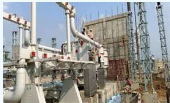
Transformer Erection Work at Inaruwa SS
