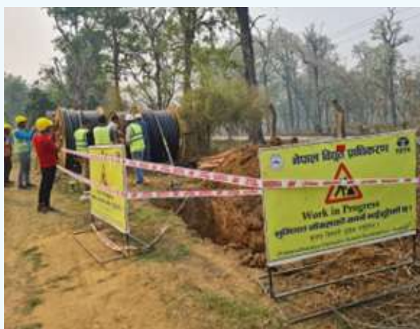
33 kV Cable Laying in Bharatpur
