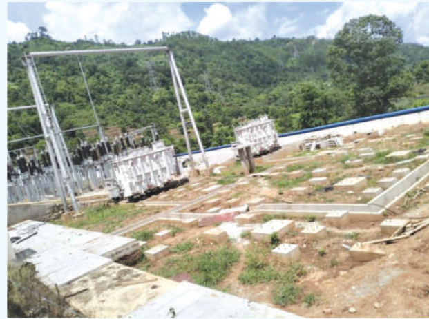
Civil Foundation at Malekhu 132 kV Switching Station
