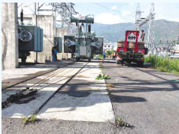
Replacement of Power Transformer at Chapali Substation
