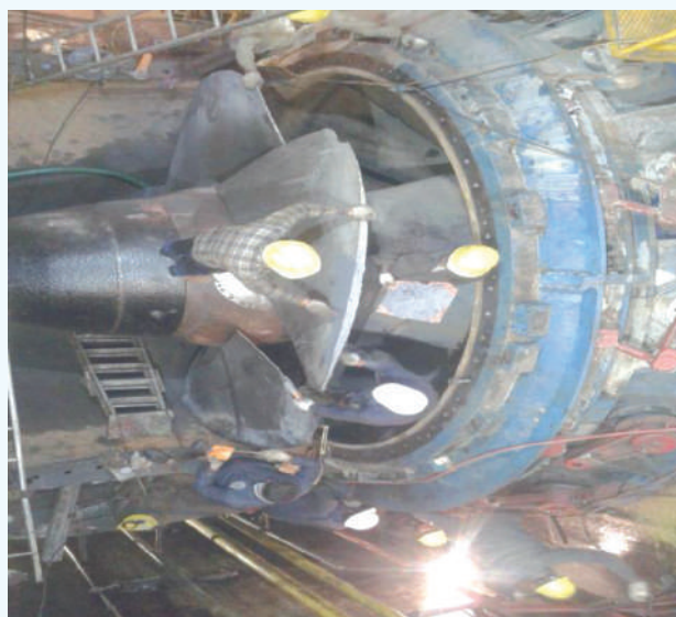
Repairing of Runner Hub and Blades
