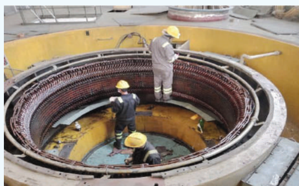
Varnishing of Generator Winding
