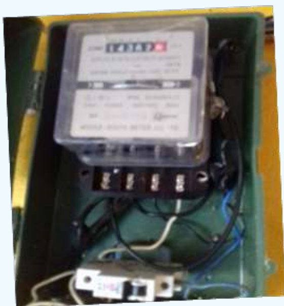
Meter Bypass in Inaruwa DC
