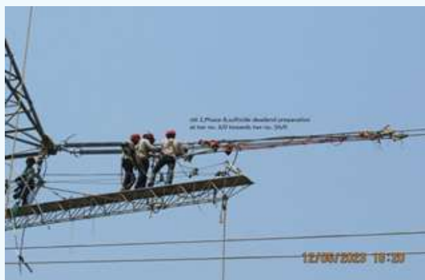
Dead End Insulator Setting of Kushma-New Butwal Line
