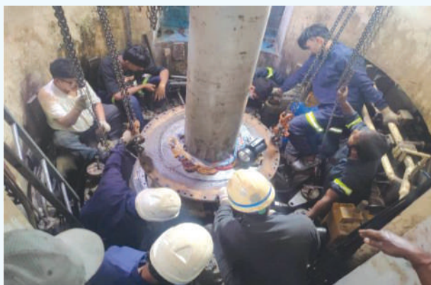
Inflatable Shaft Seal Replacement
