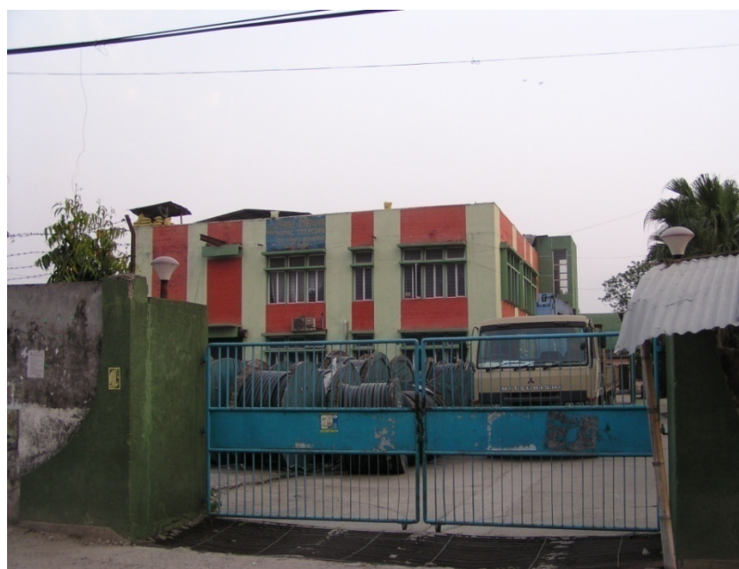
Figure 9: Nepal Telecom Building, Bharatpur
