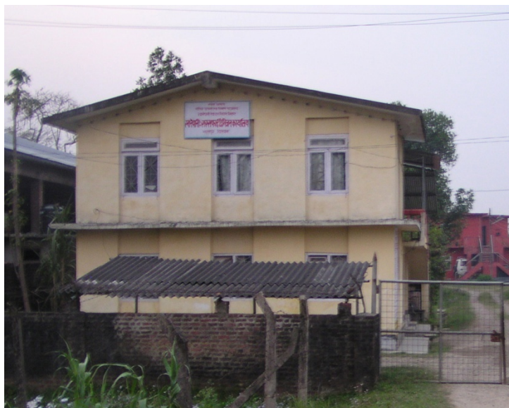
Figure 10: Nepal Water Supply Cooperation Office, Bharatpur
