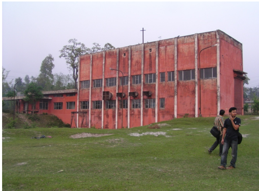
Figure 3: Narayani Lift Irrigation Pump House
