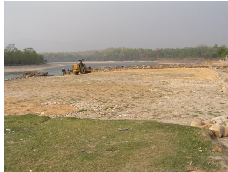
Figure 12: Under Construction Reed Bed Treatment Plant
