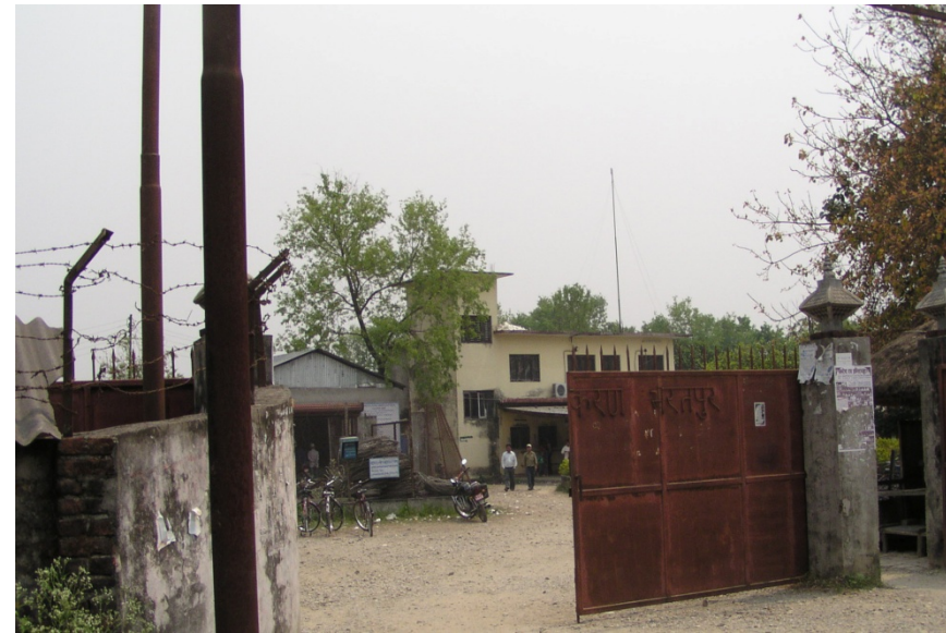
Figure 7: Nepal Electricity Authority Office, Bharatpur
