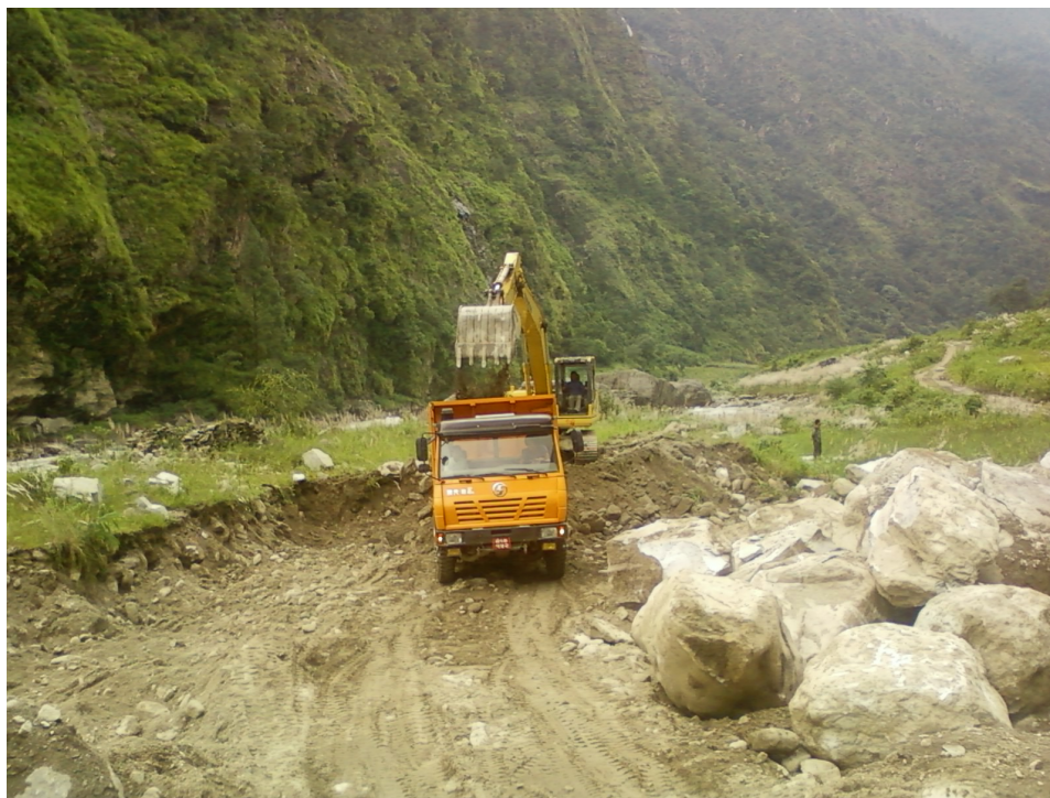
Excavation at Headworks Right Bank
