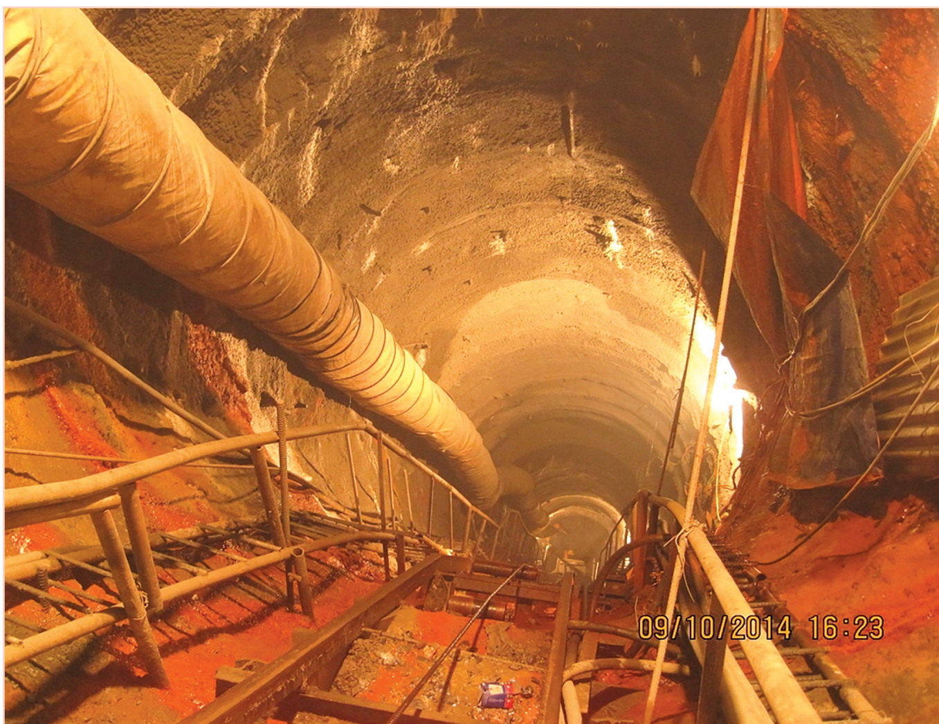
Excavation of Inclined Penstock Tunnel - Kulekhani III HEP
