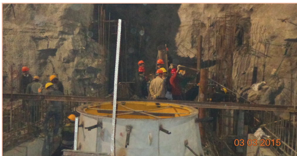
Installation of Draft Tube in Upper Trisuli-3A HEP
