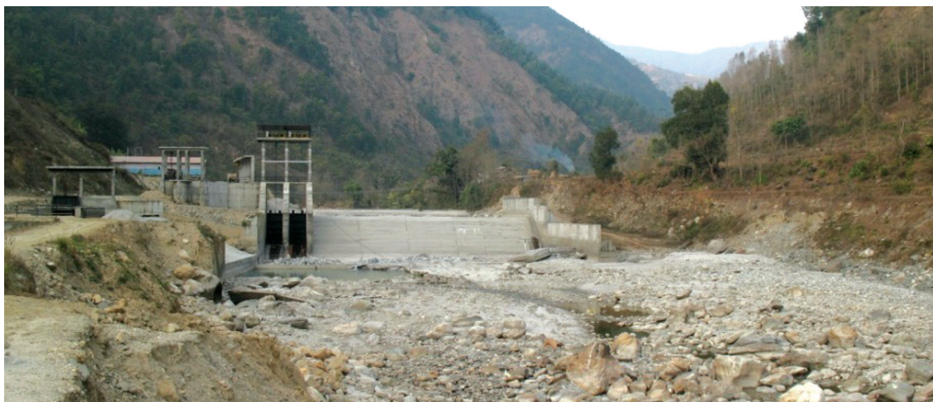
Picture 2: Dewatered stretch of Modi Khola Downstream of Modi Hydropower Project (10 MW), Parbat District (photographed: January 6, 2013)
