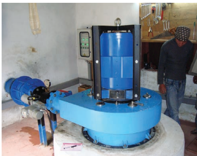
70 KW micro-hydro plant at Toktok supplying electricity to Phakding.
