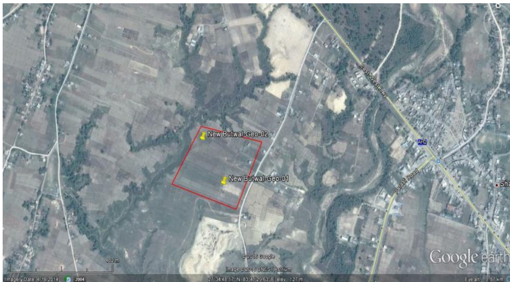
Figure 2.5.4.14: New Butwal Substation
