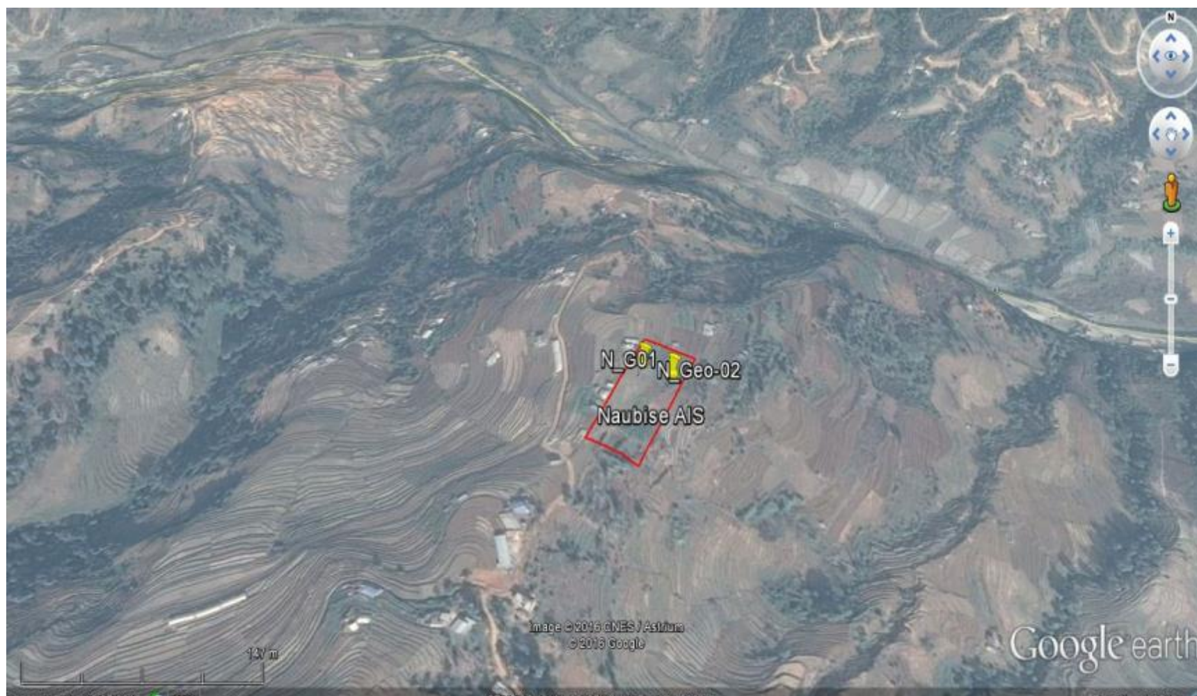
Figure 2.5.4.12 : Naubise Substation (Zoom Out)
