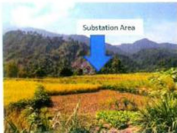
Proposed Saranghat Substation
